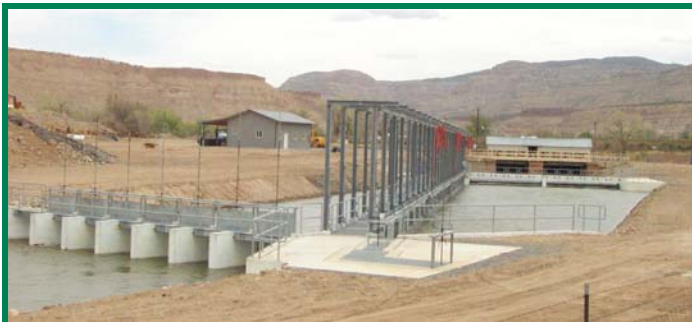
Fish Screen at Grand Valley Irrigation Company (GVIC) Diversion
