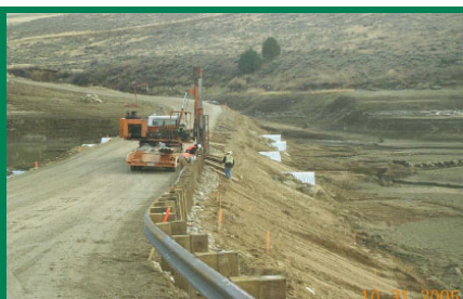
Picture 1. Detour road across the drained upper reservoir
