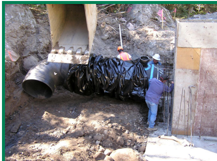
Laying 30-inch HDPE pipe at headgate
