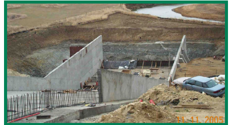
Picture 4. Splash pool for the new emergency spillway channel.
