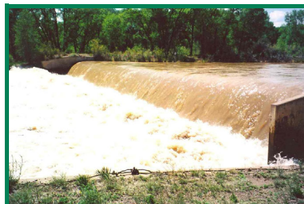
Rio Grande Canal diversion at 5000+ cfs.
