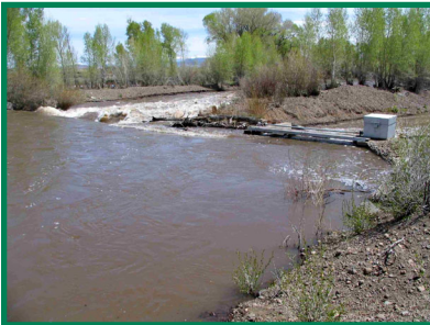
San Antonio Bifurcation almost overflowing
