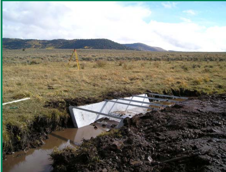
Photo 2. Completion of flume installation.
