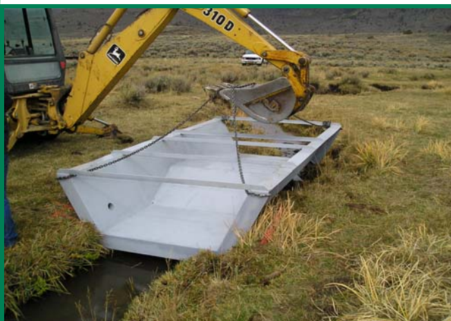
Photo 1. Tracing out where flume is to be installed.
