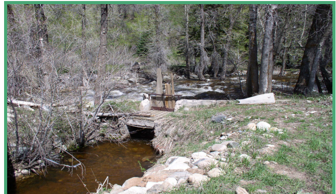
Enterprise Ditch and headgate before construction.
