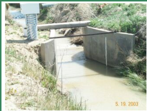
Water from the Catlin Canal measured and returned for replacement of well depletions
