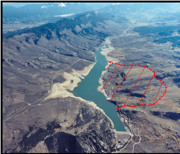
Photo taken on October 8, 2002, looking south. Heeneey and the potential slide area are highlighted. The Williams Fork range is on the left. At the time of the photo, the reservoir elevation was 7,879.21 feet; storage was 48,782 acre-feet. On September 3, 2002, Green Mountain hit its lowest elevation in 40 years at 7,875.08 feet (45,101 acre-feet).
