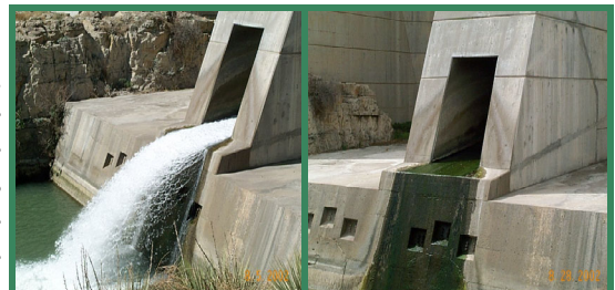
One or more gates usually are releasing water as shown on the left. In 2002, Arkansas River flows were so low that all of the main gates were shut and a small gate through the fish hatchery was used to supply most of the flow below the dam.
