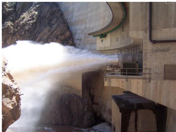
Strontia Springs Dam, Division 1
