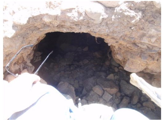
Trujillo Meadows Dam, Division 3
