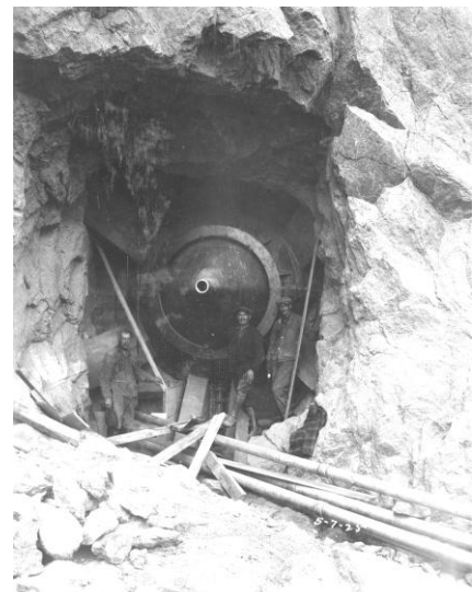
Cheesman Dam Construction – Circa 1925
