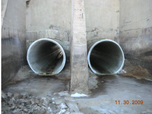
Horse Creek Dam, Division 1
