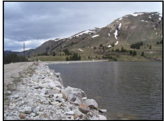
Eagle Park Dam, Eagle County High Hazard
