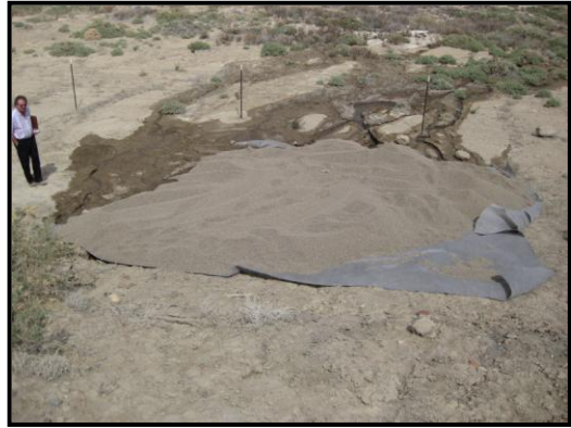
Park Center L&W # 5 Dam, Fremont County Low Hazard
