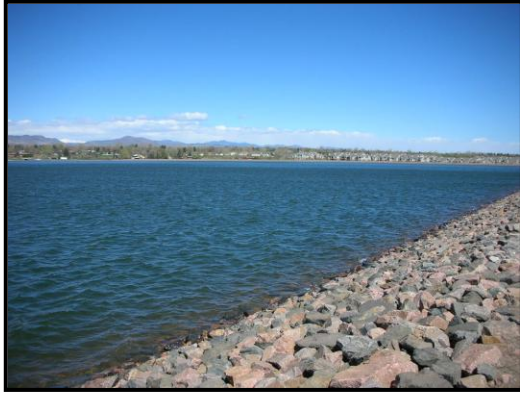
South Platte Dam, Douglas County High Hazard
