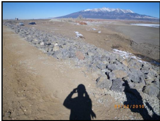
Smith Dam, Costilla County High Hazard
