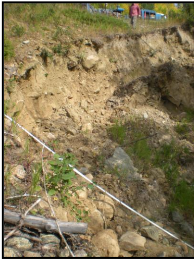
Lower Cabin Creek Dam, Clear Creek County High Hazard
