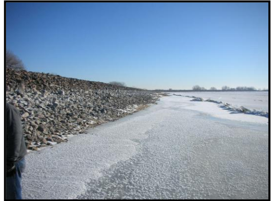
Empire Dam, Weld County High Hazard
