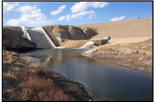
Ritschard Dam, Grand County High Hazard
