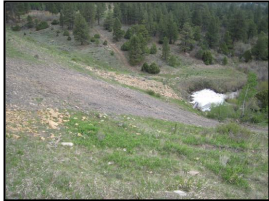
Gurley Dam, San Miguel County High Hazard
