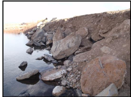
Smith Dam, Costilla County High Hazard
