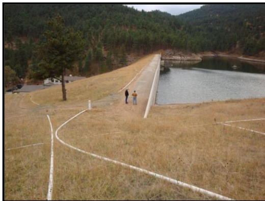
Pine Brook Dam, Boulder County High Hazard
