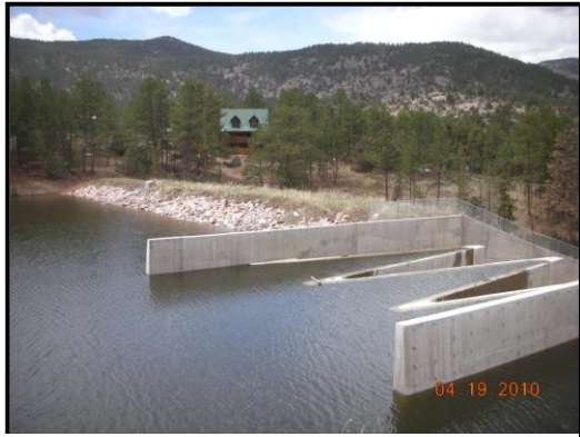
Crowlane No. 2 Dam, Larimer County High Hazard
