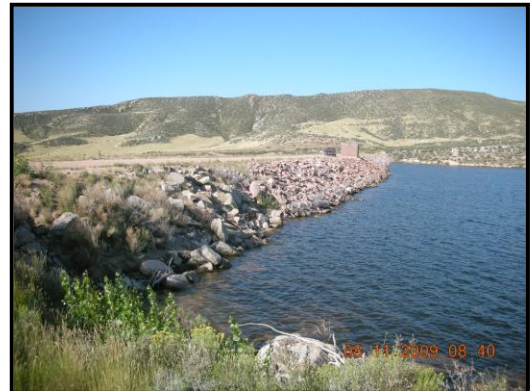
Park Creek Dam, Larimer County High Hazard
