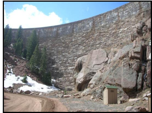
Cheesman Dam, Jefferson County High Hazard
