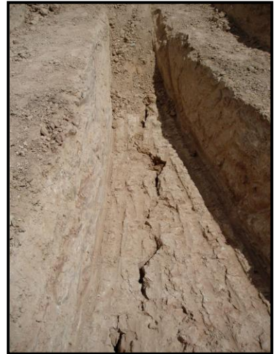
Totten Dam Montezuma County, High Hazard
