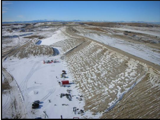
Rueter-Hess Dam, Douglas County High Hazard
