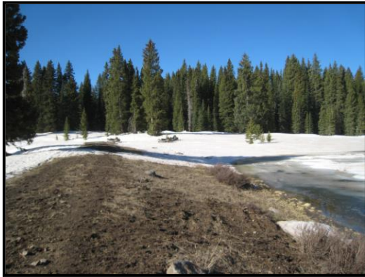
Womack #2/3 Dam, Delta County Low Hazard
