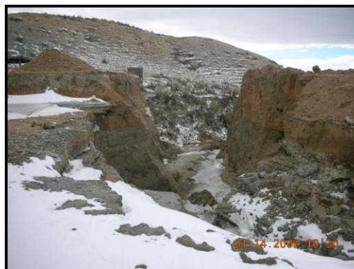
Park Creek # 2 Dam, Larimer County Low Hazard
