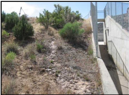
Jerry Creek # 2 Dam, Mesa County High Hazard
