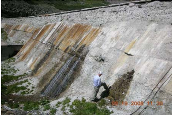
Albion Lake Dam, Boulder County Division 1, Significant Hazard
