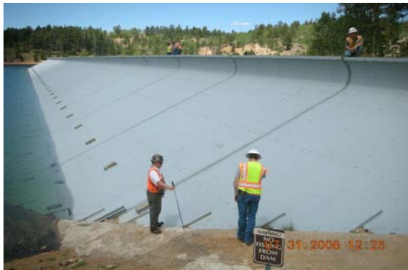
South Catamount, Teller County Division 2, High Hazard
