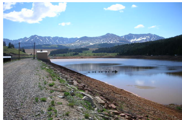
Robinson Dam, Summit County Division 5, High Hazard
