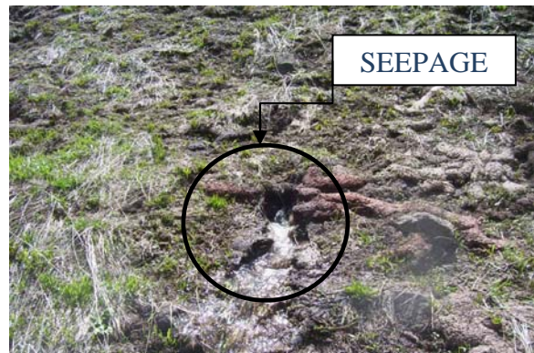
Hopkins Dam, Garfield County Division 6, Significant Hazard
