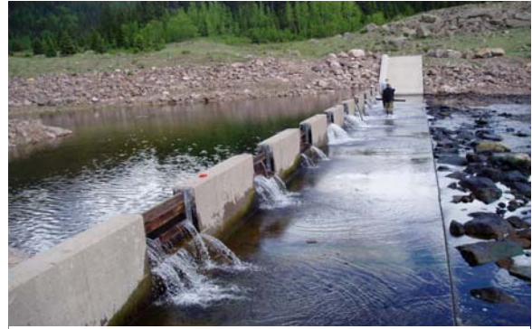
Trujillo Meadows Dam, Conejos County Division 3, Significant Hazard
