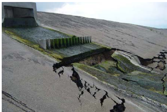
Bull Canal Dam, Weld County Division 1, High Hazard
