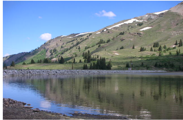
Eagle Park Dam, Eagle County Division 5, High Hazard
