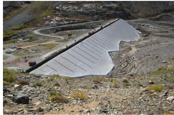
Upper Blue Dam, Summit County Division 5, High Hazard
