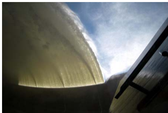
Crystal Dam, Montrose County Division 4, High Hazard
