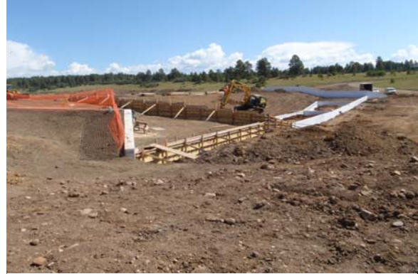
Stevens Dam, Archuleta County Division 7, Significant Hazard
