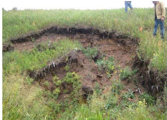
Green Valley Retention Dam, Jefferson County Division 1, Low Hazard
