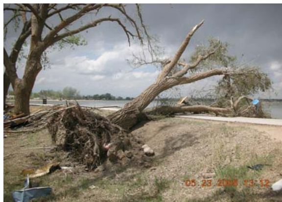
Windsor Lake Dam, Weld County Division 1, High Hazard
