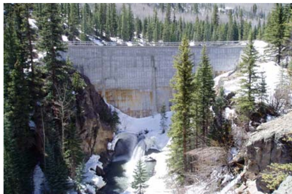
Humphreys Dam, Mineral County Division 3, High Hazard
