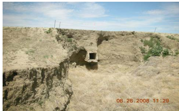
Jolly John Dam, Arapahoe County Division 1, Low Hazard
