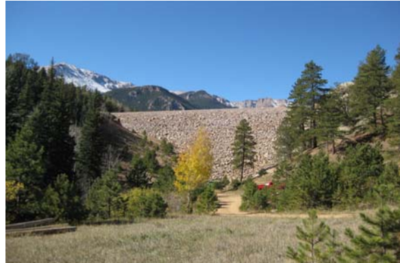
Manitou Dam, El Paso County Division 2, High Hazard
