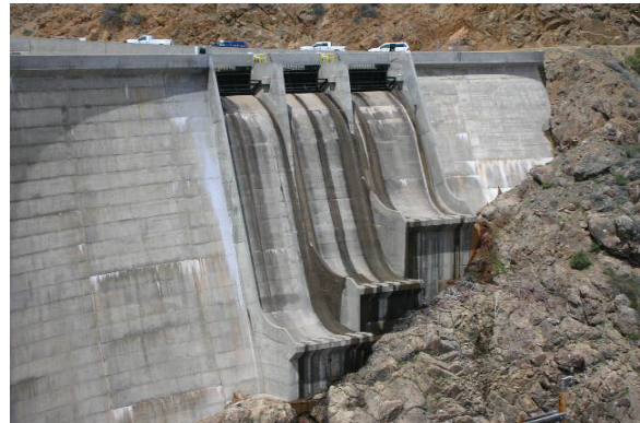
Williams Fork Dam, Grand County Division 5, High Hazard
