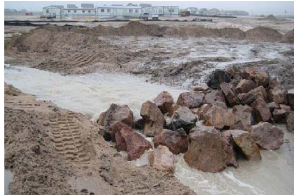
Sand Creek Detention Dam, El Paso County Division 2, Non Roster
