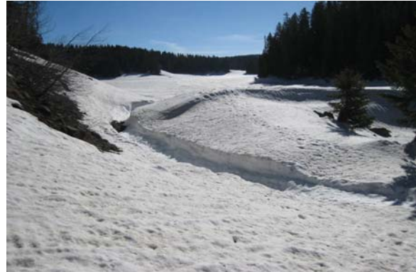
Donnelly #1 Dam, Delta County Division 4, Significant Hazard
