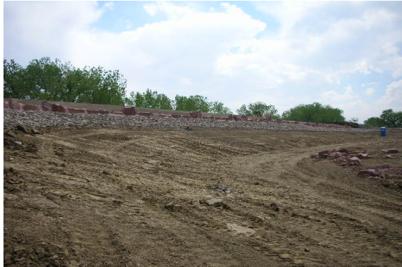
Margaret-Carpenter Dam, Adams County Division 1, Low Hazard
