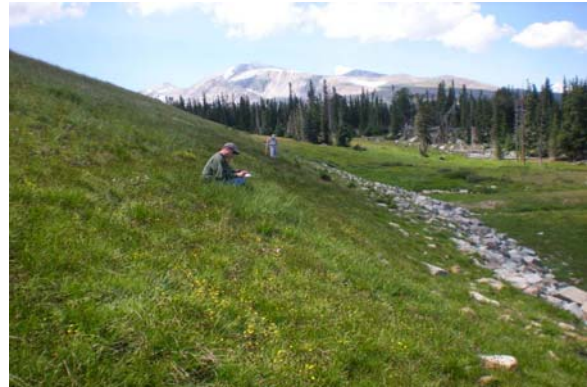
Left Hand Park Dam, Boulder County Division 1, High Hazard
