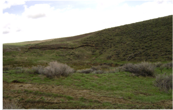
Biskup Dam, Moffat County Division 6, Low Hazard
