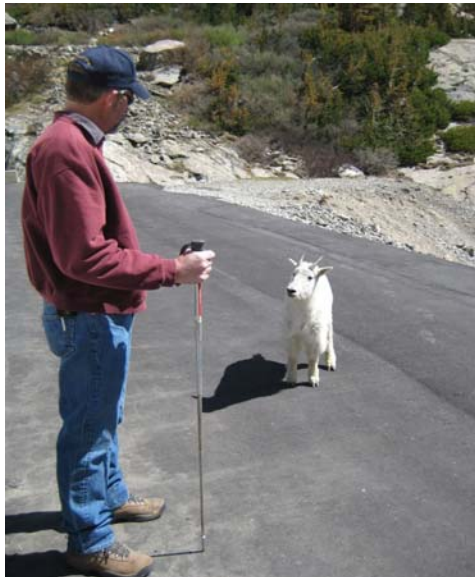
Upper Blue Dam, Summit County, Division 1, High Hazard
