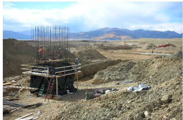
James Tingle Dam, Park County Division 1, High Hazard
