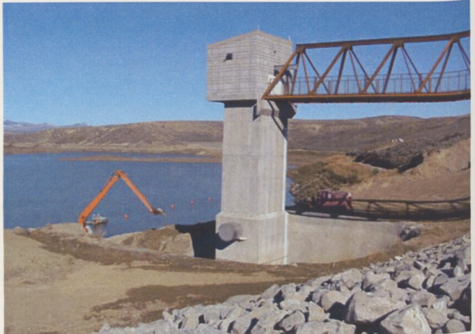
Elkhead Dam Outlet Works Tower Moffat County, Division 6, High Hazard
