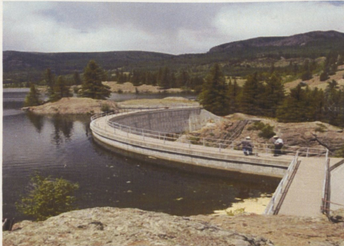
Humphreys Dam, Mineral County Division 3, High Hazard
