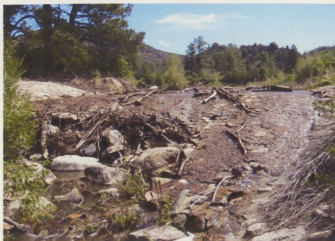
Keeton Dam, Emergency Spillway, El Paso County, Division 2, Low Hazard
