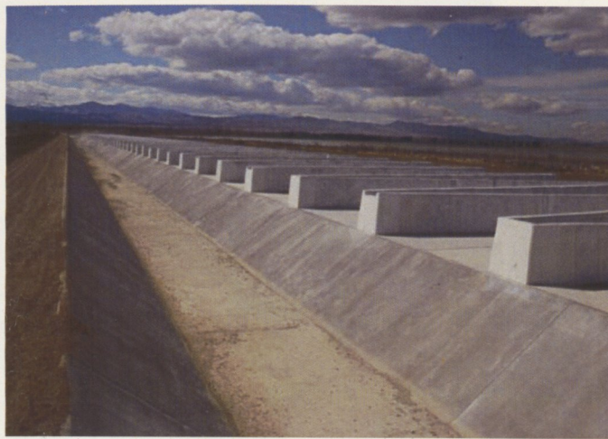
Boyd Lake, Labyrinth Spillway Larimer County, Division 1, High Hazard
