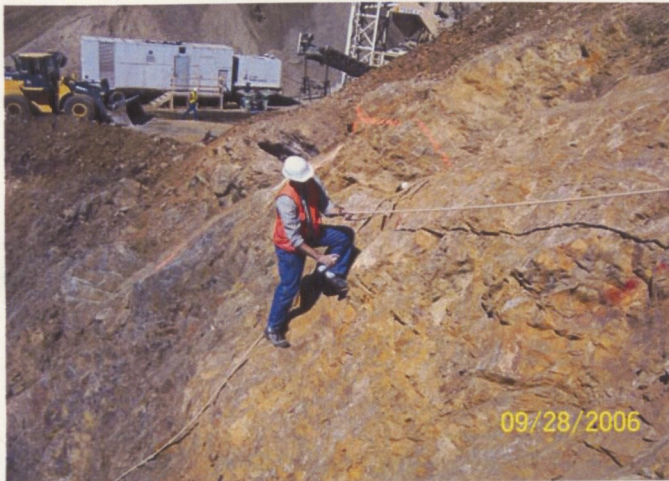
Genesee Dam No. 2 Foundation Inspection, Jefferson County, Division 1, High Hazard
