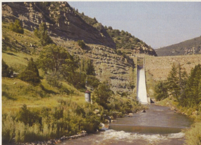
Paonia Dam, Gunnison County Division 4, High Hazard
