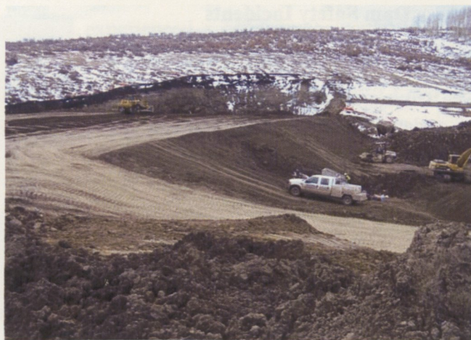
Cornerstone Pond No. 4 Construction Ouray County, Division 4, Significant Hazard
