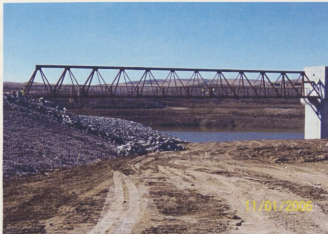
Elkhead Dam, Moffat, County Division 6, High Hazard
