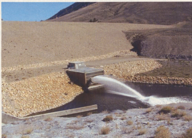
Ritschard Dam, Grand County Division 5, High Hazard
