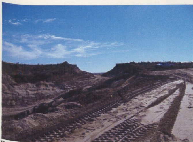
Prewitt Dam Emergency Spillway Construction Washington County, Division 1, High Hazard
