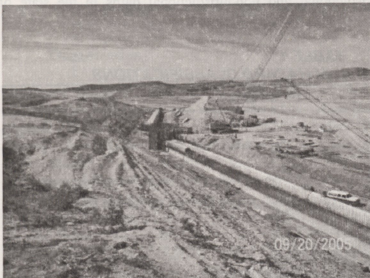
Outlet works construction at Rueter-Hess Dam
