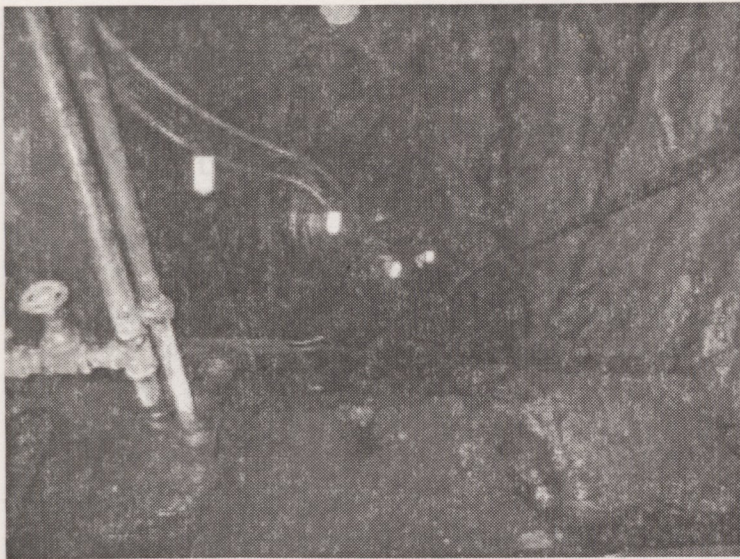
Interior of Cheesman Dam Outlet Works (carved within solid granite)
