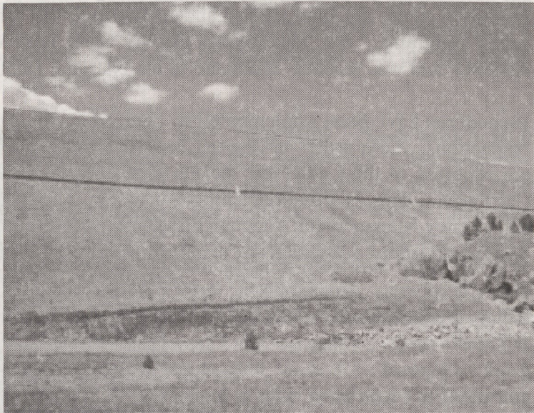
Downstream slope of Rampart Dam, a 220 foot-tall earth dam.
