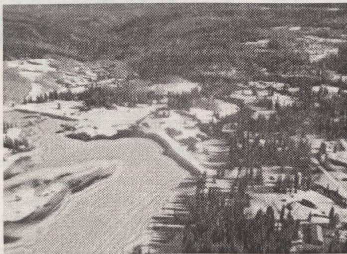
Aerial view of Bonham Reservoir dikes in May
