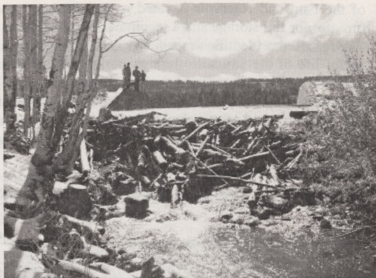
Mesa Creek #1 Dam spillway during spring runoff
