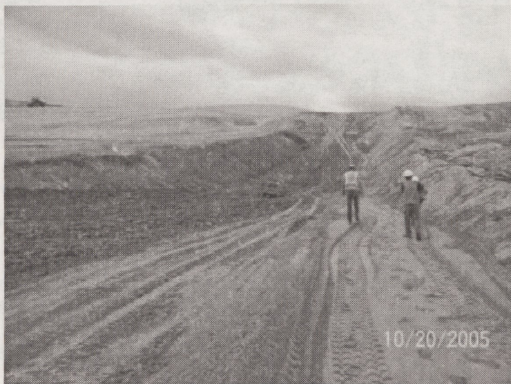
Core trench fill and chimney drain installation at Rueter-Hess Dam.
