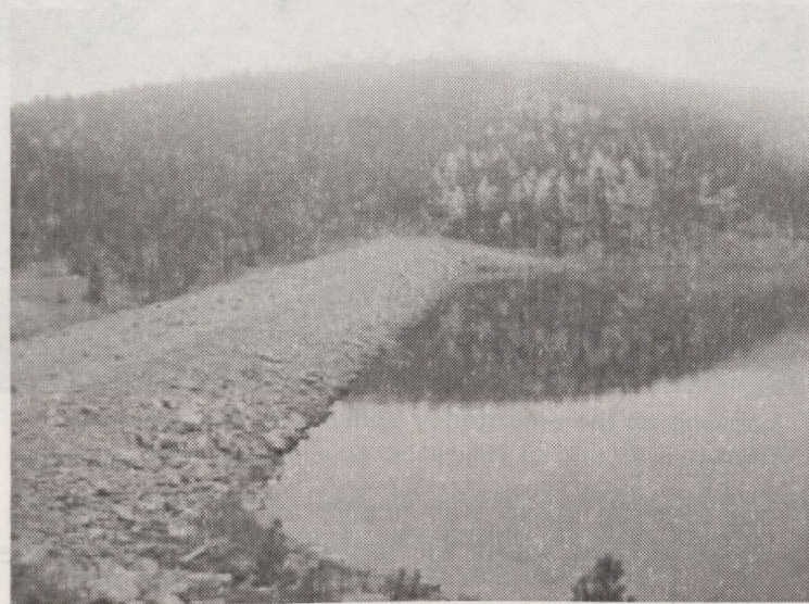
The upstream face of Manitou Dam during the Fall annual inspection.
