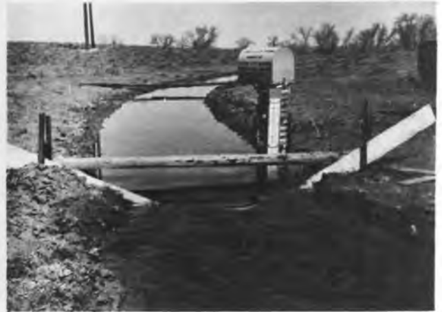
Photo 2. Upstream gaging station with triangular weir and recorder.
