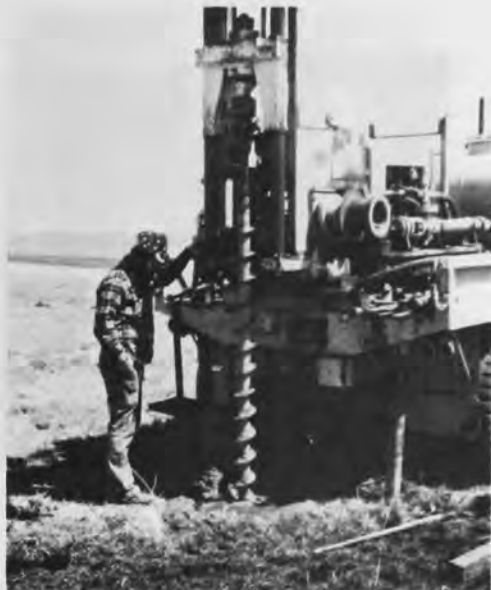
Photo 3. Drilling rig used to install observation and recorder wells.
