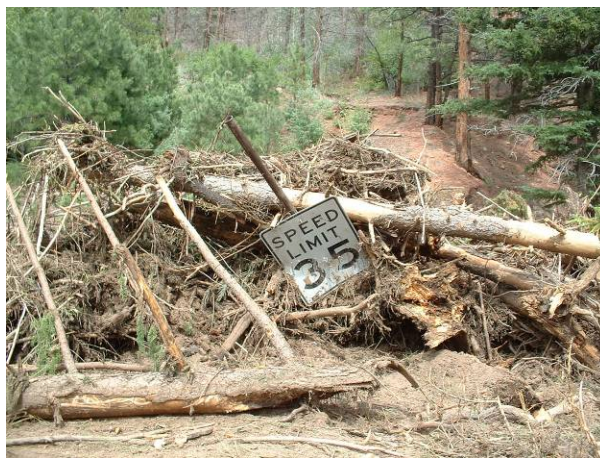
Figure 2.38 – West Creek – Highway 67 Road Damage
