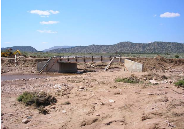
Figure 1.31 – County Road 123 Bridge – Eightmile Creek Bridge Overtopping, Downstream Face
