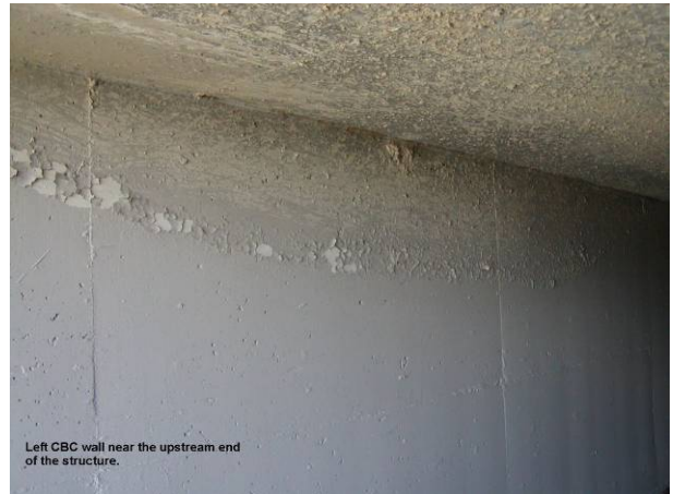
Figure 3.13 – Bosley Wash – I-70 Culvert Highwater Marks
