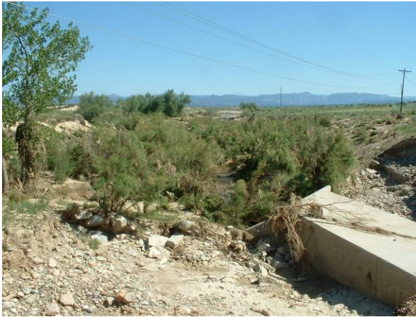
Figure 1.20 – Brush Hollow Creek - Highway 115 Culvert Looking Upstream
