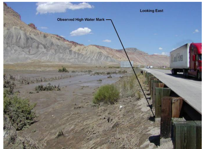
Figure 3.7 – Bosley Wash – I-70 Culvert looking east along north side of road.
