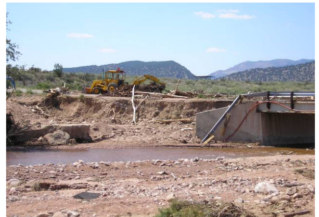
Figure 1.34 – County Road 123 at Eightmile Creek, Downstream Wing-wall
