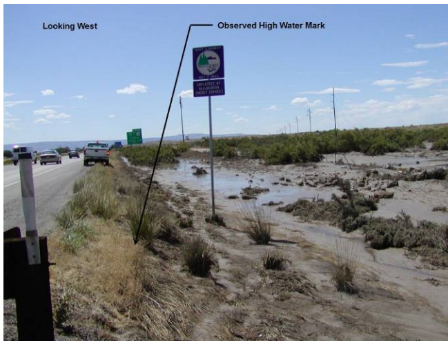
Figure 3.6 – Bosley Wash – I-70 Culvert looking west along north side of road.
