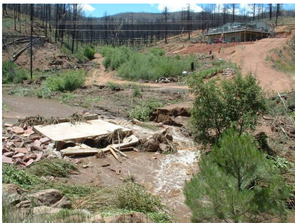
Figure 2.35 – West Creek – Private Road Crossing. Note proximity of Hayman burn.
