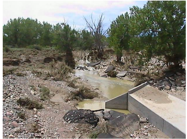
Figure 1.21 – Brush Hollow Creek - Highway 115 Culvert Looking Downstream
