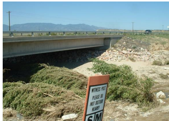
Figure 1.27 – Brush Hollow Creek Highway 50 Bridge – Eastbound Bridge Note: no reported overtopping.
