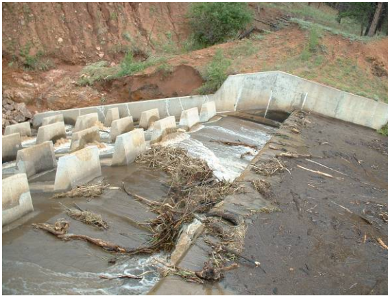
Figure 2.19 – West Creek – J.O. Hill Reservoir Emergency Spillway
