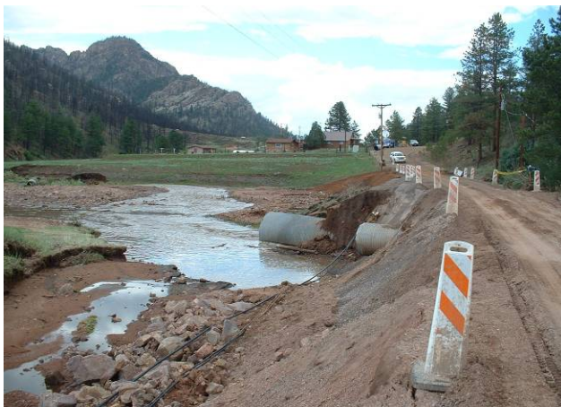
Figure 2.25 – West Creek – Abbey Road Crossing
