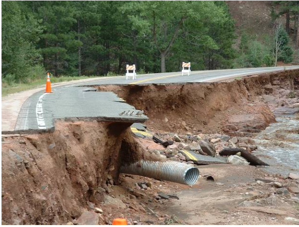
Figure 2.27 – West Creek - Highway 67 Culvert Looking Upstream
