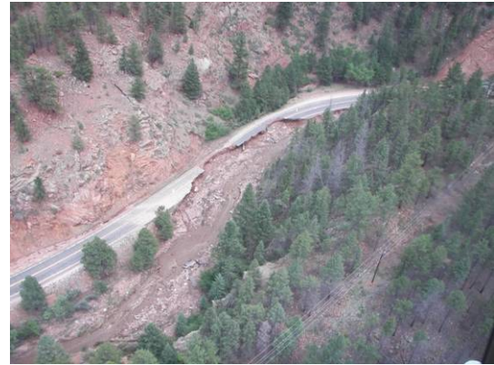
Figure 2.28 – West Creek - Highway 67 Shoulder Damage Photo courtesy of CDOT
