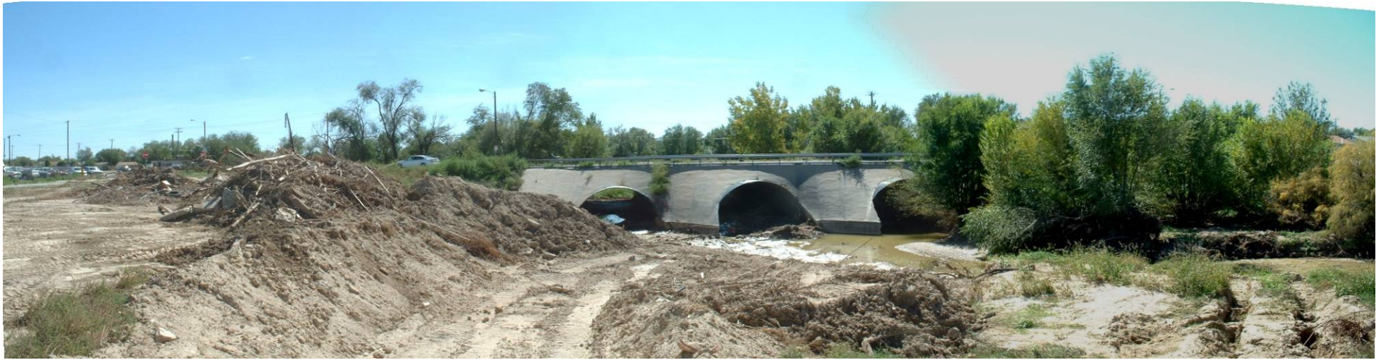
Figure 4.18 – Upstream Panoramic Picture of 18 th Street Bridge at Wild Horse Creek
