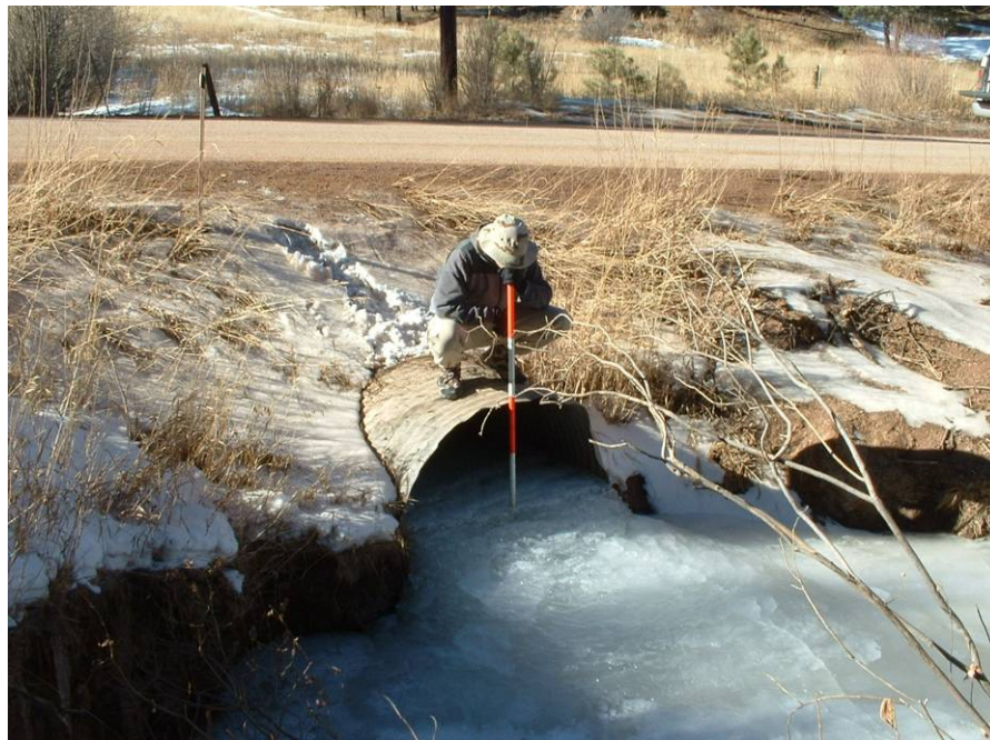
Figure 2.18 – Picture of Abbey Avenue Crossing Along West Creek before July 7, 2006 Flood Picture courtesy of Moser and Associates Engineering
