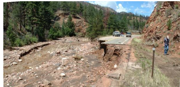
Figure 2.28 – West Creek - Highway 67 Shoulder Damage Photo courtesy of CDOT
