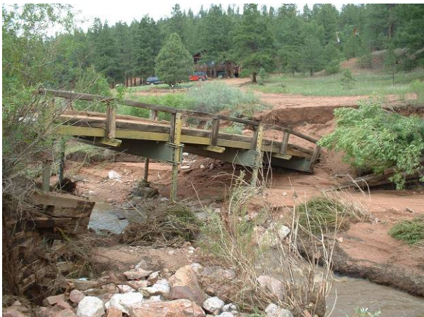
Figure 2.21 – West Creek – Private Bridge Downstream of J.O. Hill Reservoir
