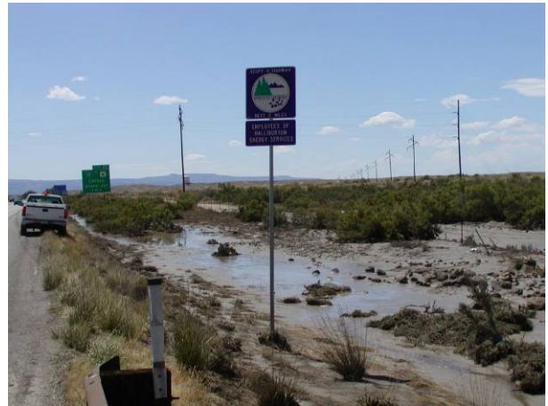
Figure 3.11 – Bosley Wash – I-70 Ponding along northern edge of roadway
