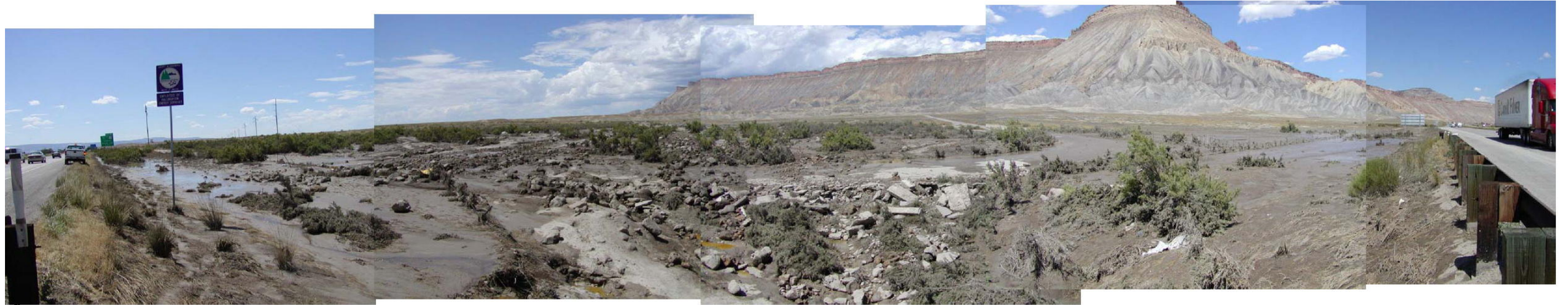
Figure 3.14 – Panorama picture looking upstream of I-70 Culvert
