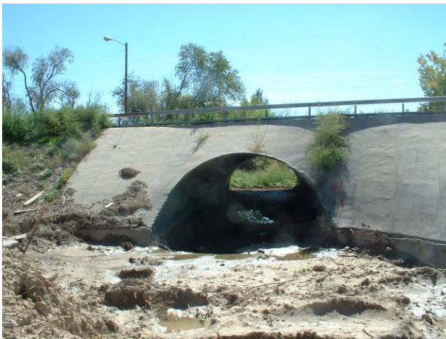
Figure 4.16 – 18 th Street Bridge – Eastern Culvert at Wild Horse Creek
