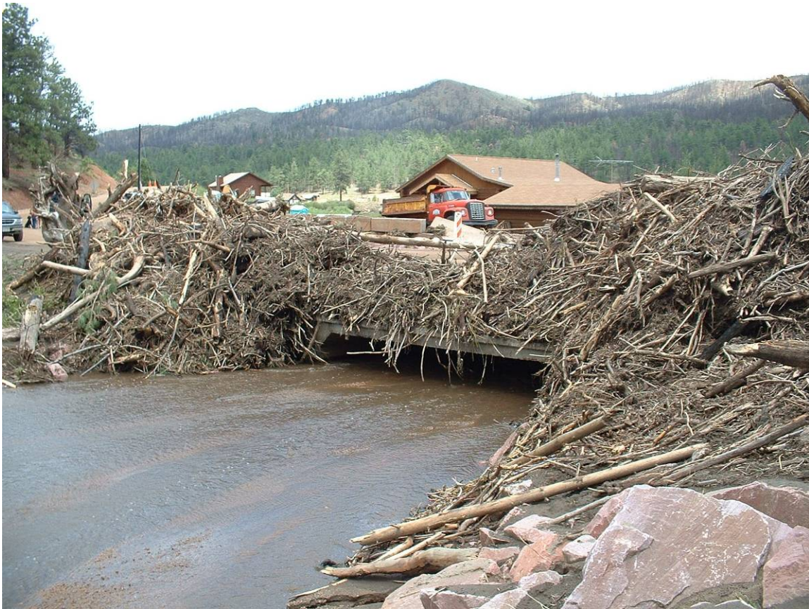
Figure 2.44 – Picture Taken from Upstream of Box Culvert at Road Crossing on July 11 th
