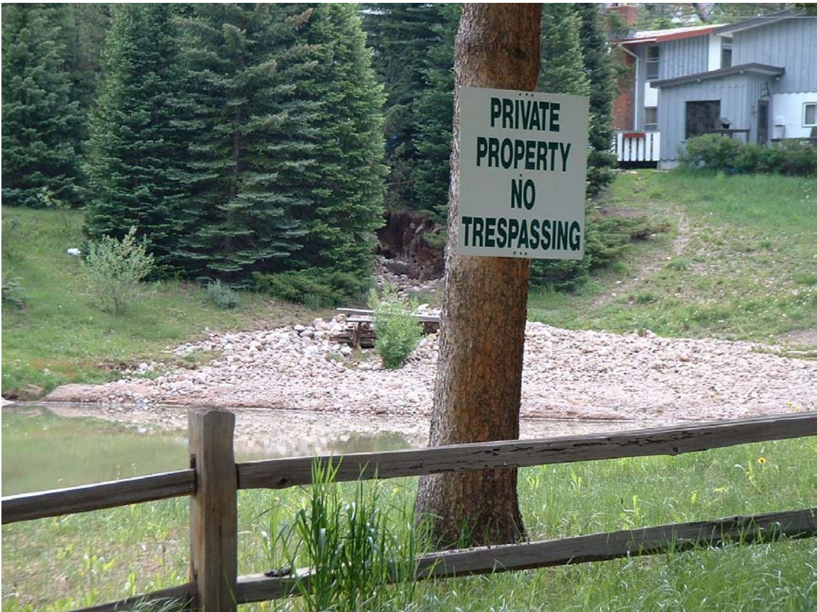
Figure 1.30 –Picture of Debris Pile at Pond near Columbine Drive after the Storm Courtesy of Site Visit by ICON Engineering, Inc.
