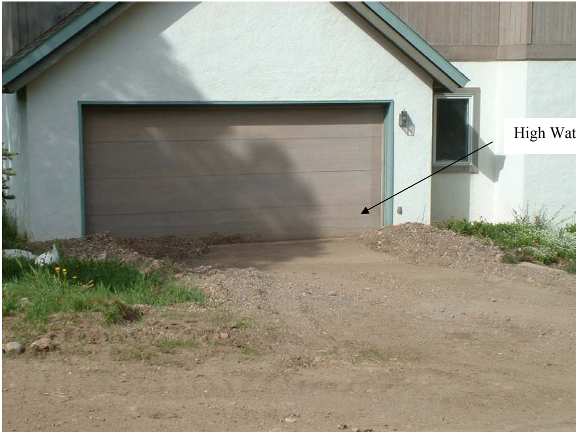
Figure 1.31 – Picture of Debris Piles and High Water Mark on Residence along Spruce Way Courtesy of Site Visit by ICON Engineering, Inc.
