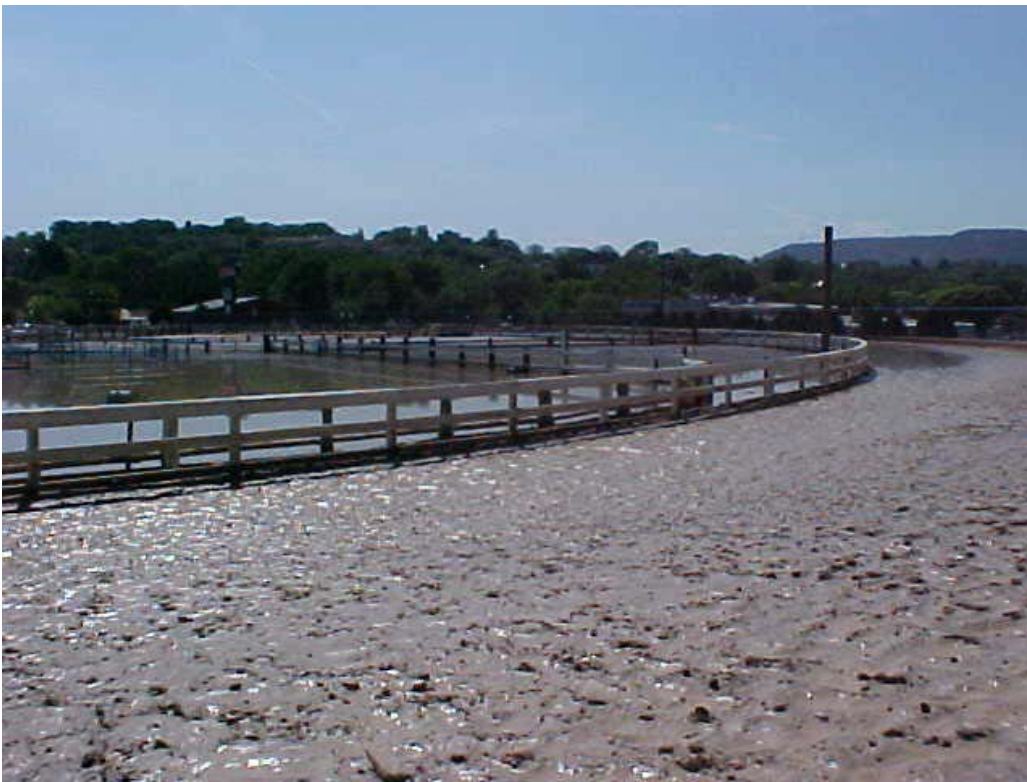
Figure 2.14 – Rifle Fairgrounds Damage Picture 4.
