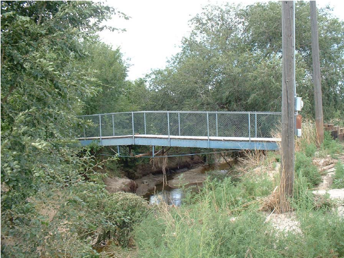
Figure 6.23 – Walking Bridge Over Wiley Drainage Ditch on September 3, 2002.
