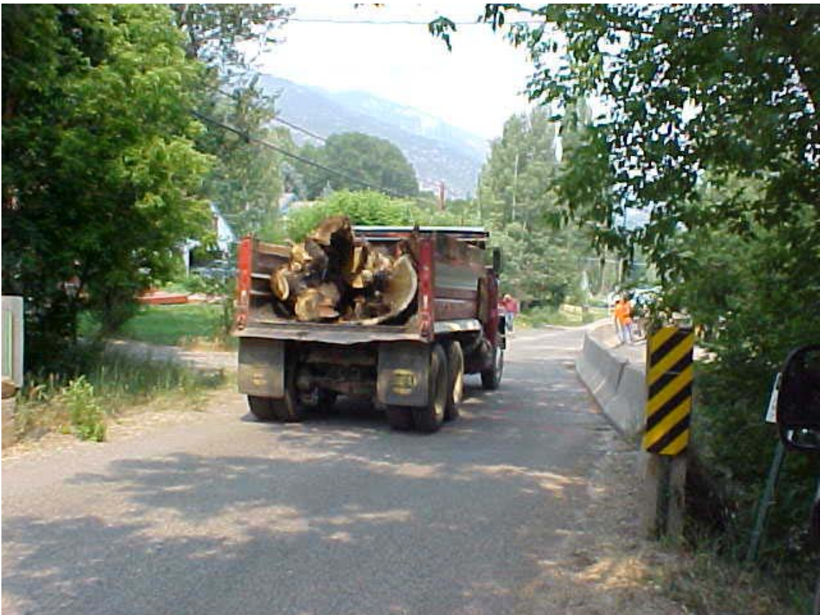
Figure 5.20 – Picture of Dump Truck with Typical Debris Being Removed During Mitigation Effort.
