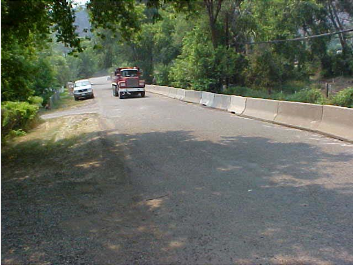
Figure 5.21 – Picture of Donagan Road with Jersey Barriers Installed During Mitigation Effort.
