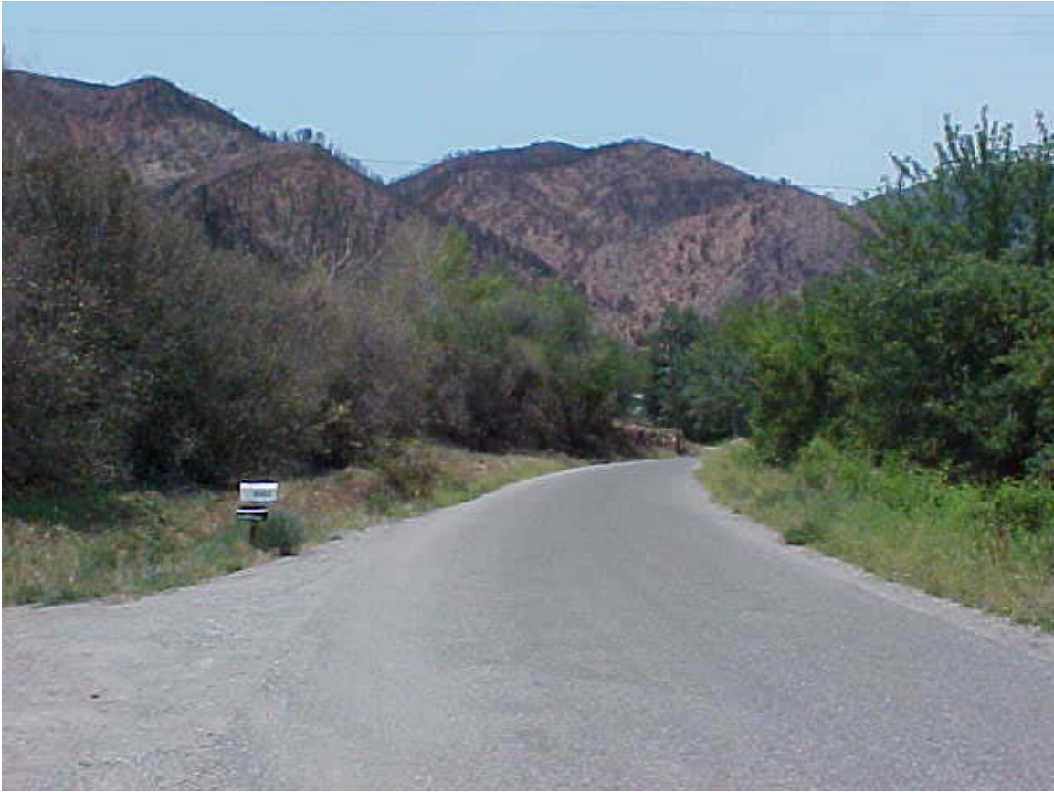
Figure 5.19 – Picture of Mitchell Creek Road Looking West During Mitigation Effort.
