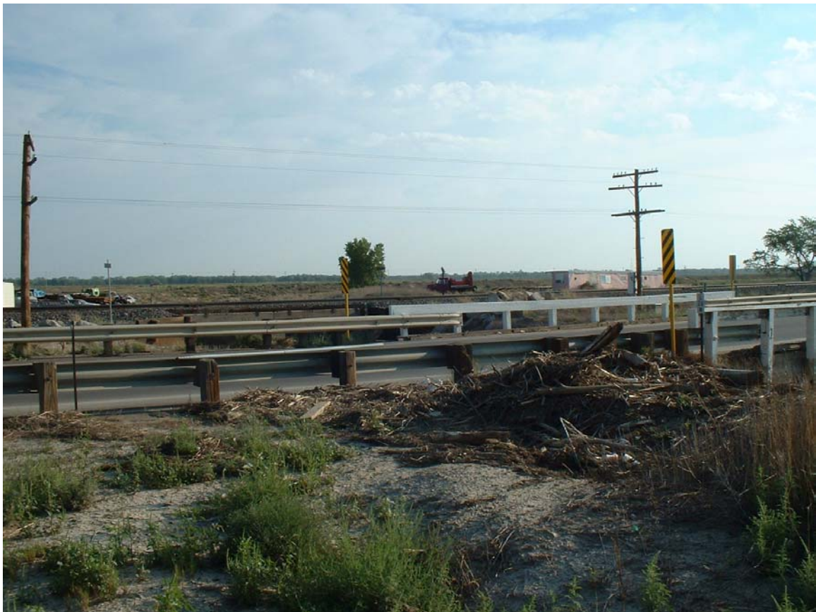
Figure 6.30 – Looking North at Debris Pile along Highway 50 in Lamar, Colorado.
