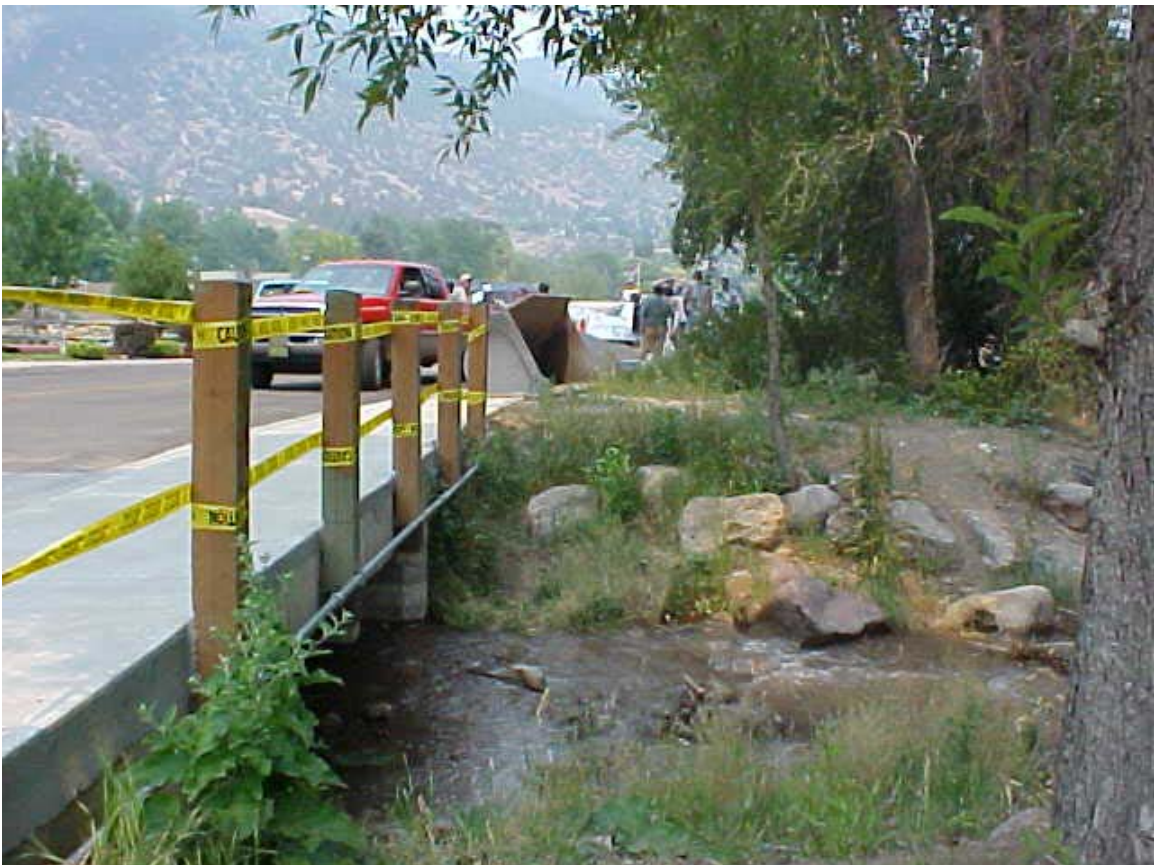
Figure 5.18 – Picture #2 of Center Street Bridge Over Mitchell Creek During Mitigation Effort.
