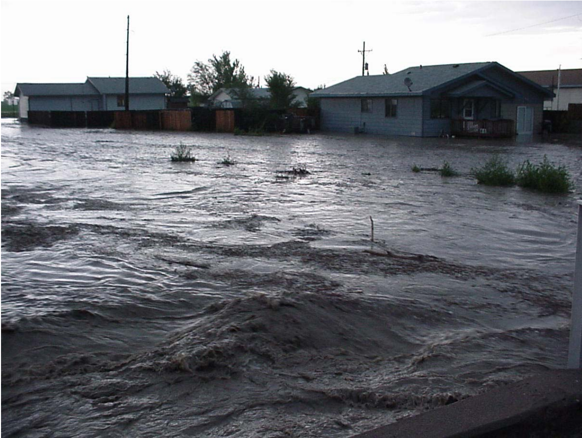
Figure 6.19 – View of Wiley Drainage Ditch from Highway 196 Bridge on August 28, 2002.
