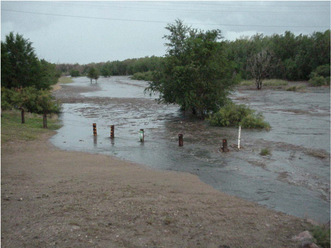
Figure 6.27 – Willow Creek Looking Downstream on August 28, 2002.
