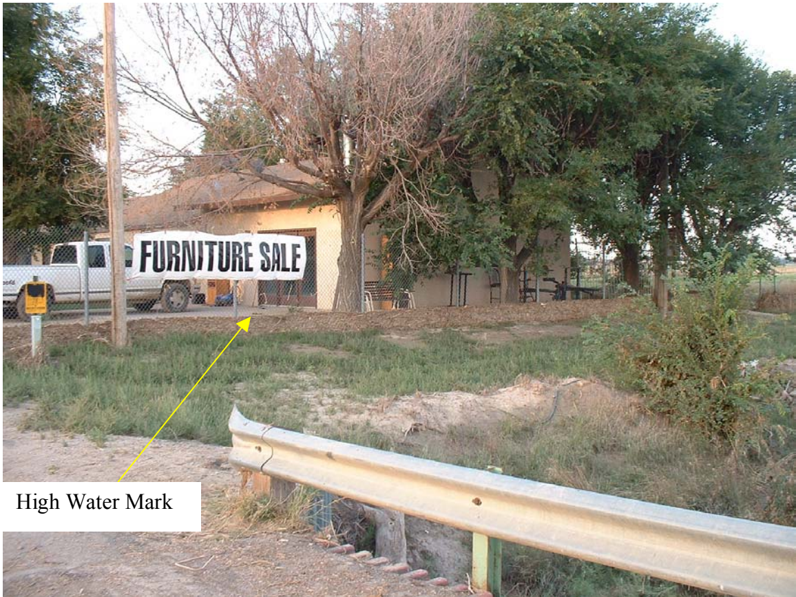
Figure 6.29 – High-Water Debris Line in Chain-Link Fence along Highway 50 in Lamar.
