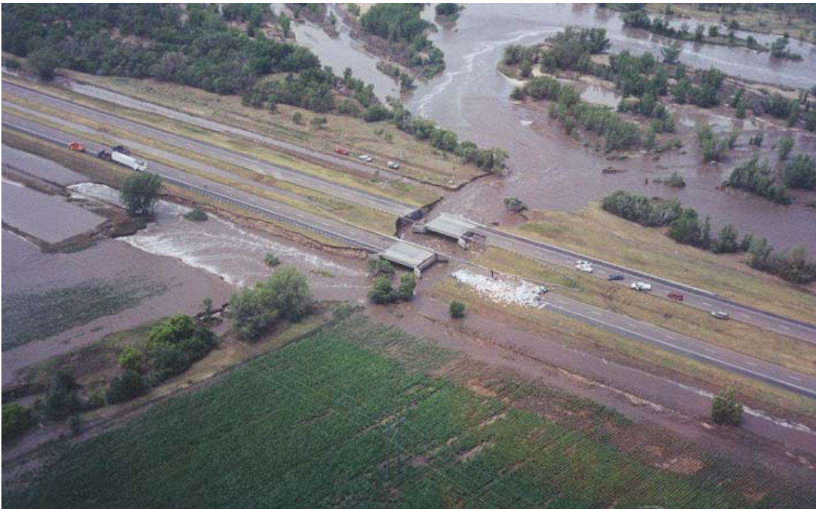
Figure 7.23 – Aerial Picture of Rural Flood Damage to Two Bridges on I-80. Picture courtesy of the Nebraska DOT.
