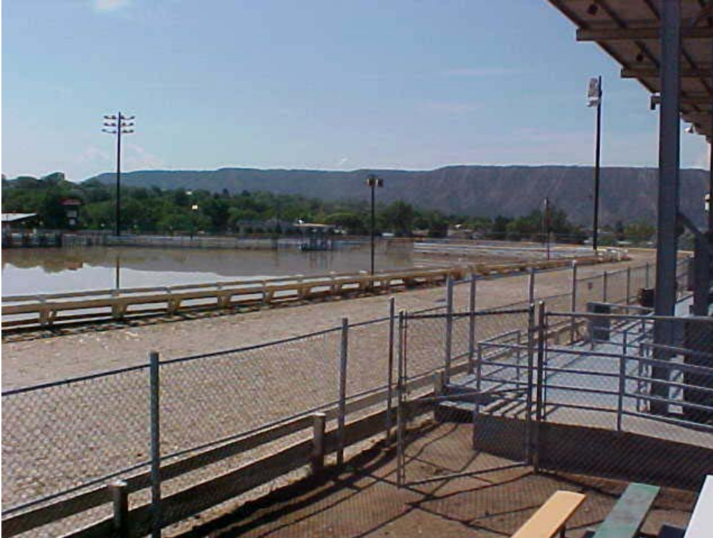
Figure 2.13 – Rifle Fairgrounds Damage Picture 3.
