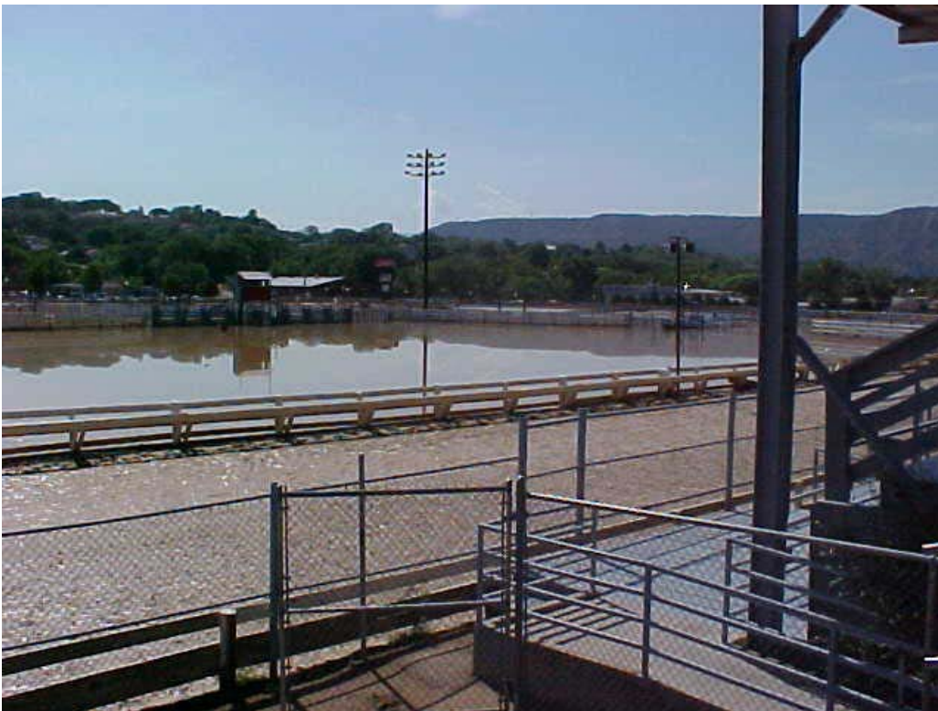
Figure 2.12 – Rifle Fairgrounds Damage Picture 2.
