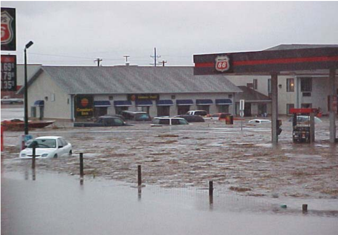
Figure 7.26 – Local Business Flooding Due to July 6 th Event. Picture courtesy of the Nebraska DOT.
