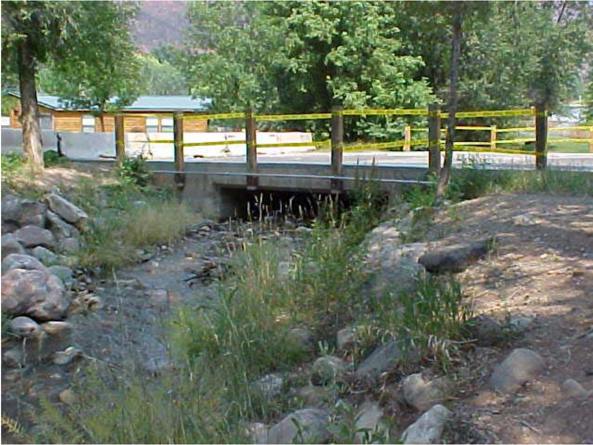
Figure 5.17 – Picture of Center Street Bridge Over Mitchell Creek During Mitigation Effort.
