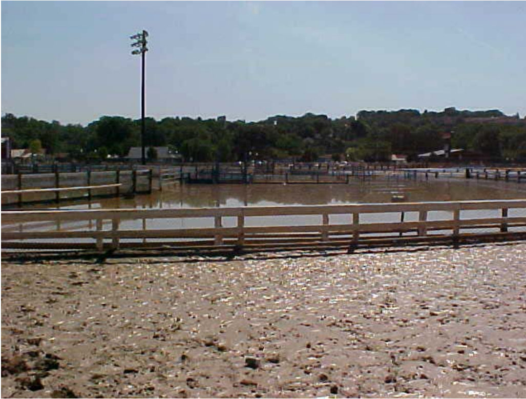
Figure 2.15 – Rifle Fairgrounds Damage Picture 5.
