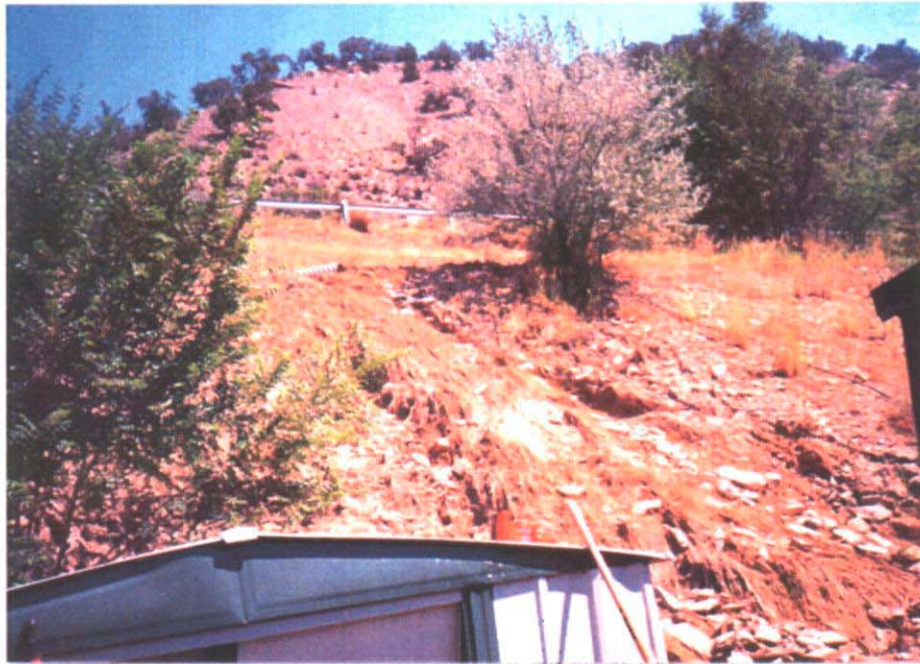
Further examples of residential flood damage in the City of New Castle
