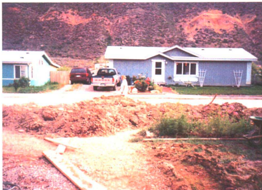
Further examples of residential flood damage in the City of New Castle
