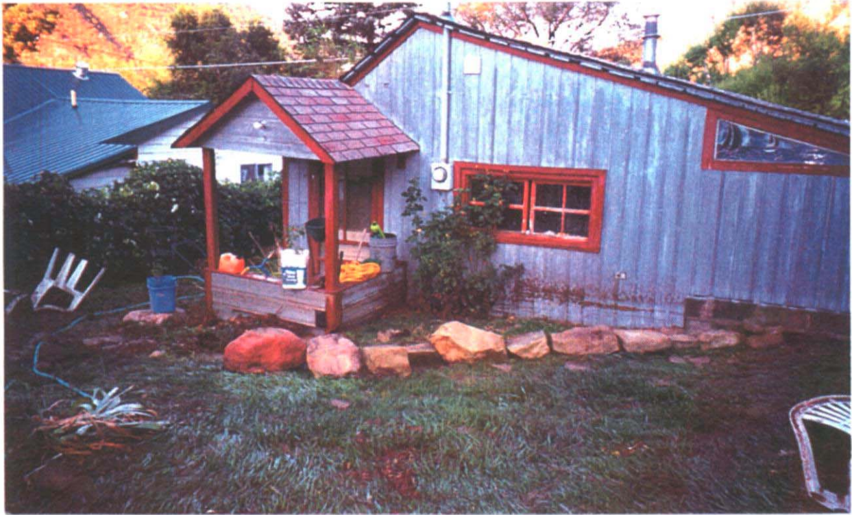
Example of residential flood damage in the City of New Castle
