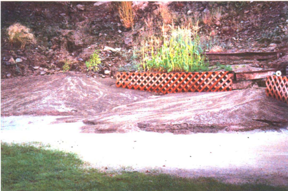
Further examples of residential flood damage in the City of New Castle
