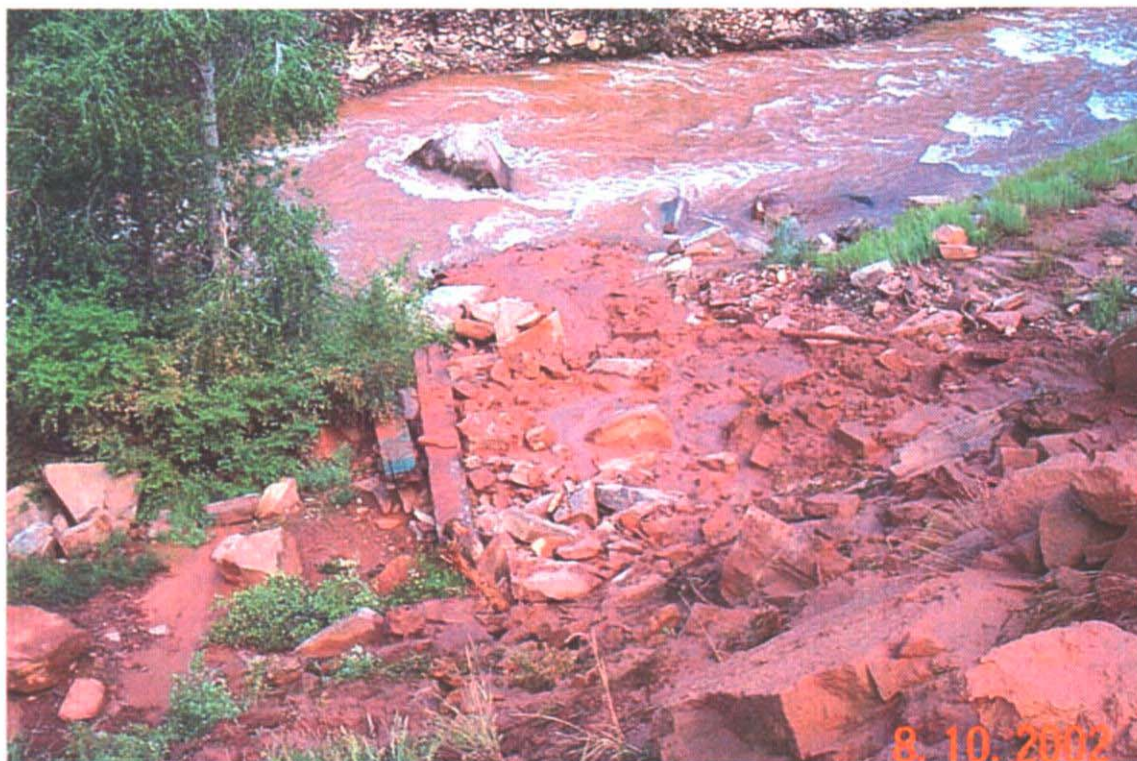
Examples of embankment drainage into the San Miguel River – Telluride vicinity
