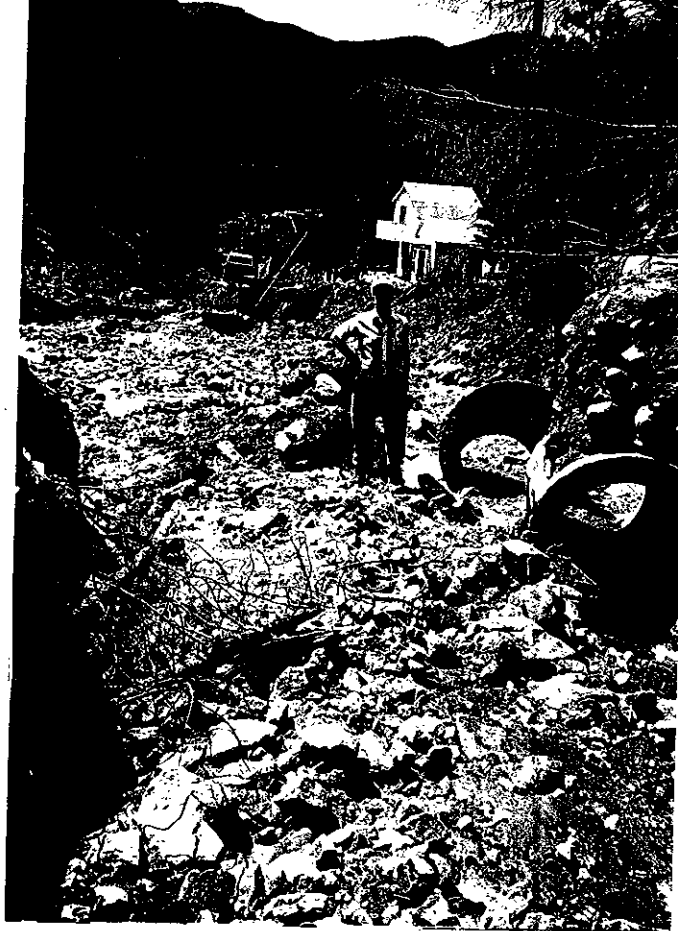
Undermined Culverts and Debris Flow on Virginia Canyon Creek - August 2, 1994
