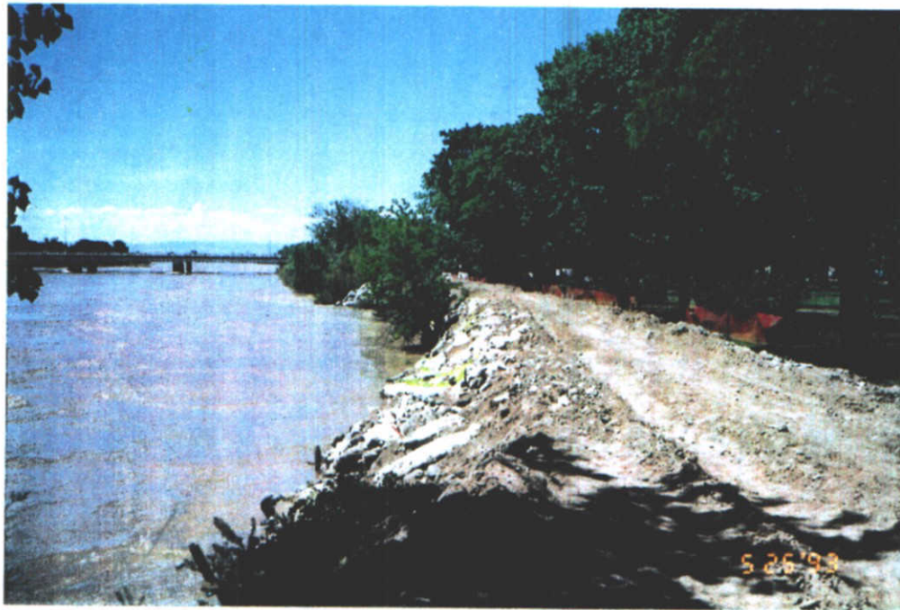
Emergency Levee at Riverside Subdivision - Grand Junction, CO
