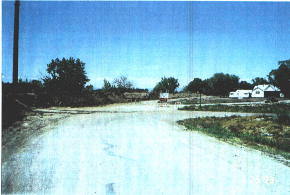
Emergency Levee at Riverside Area in Grand Junction, CO
