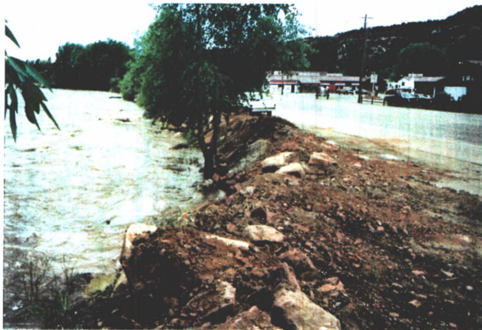
Non-Engineered Levee at Dolores, Colorado on the Dolores River
