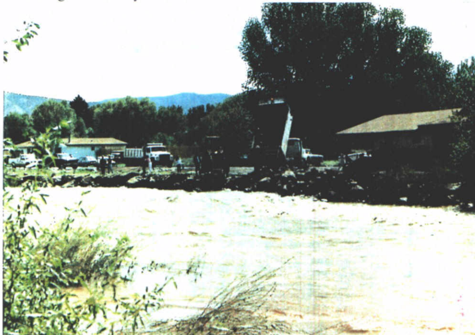
Emergency Bank Stabilization Operations at Paonia, Colorado
