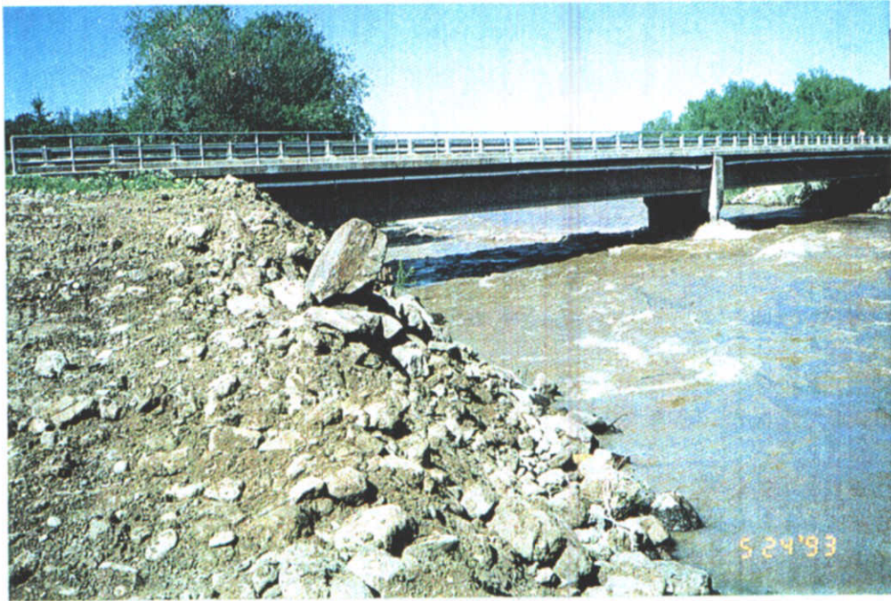
Emergency Bridge Abutment Protection - Delta County, Colorado
