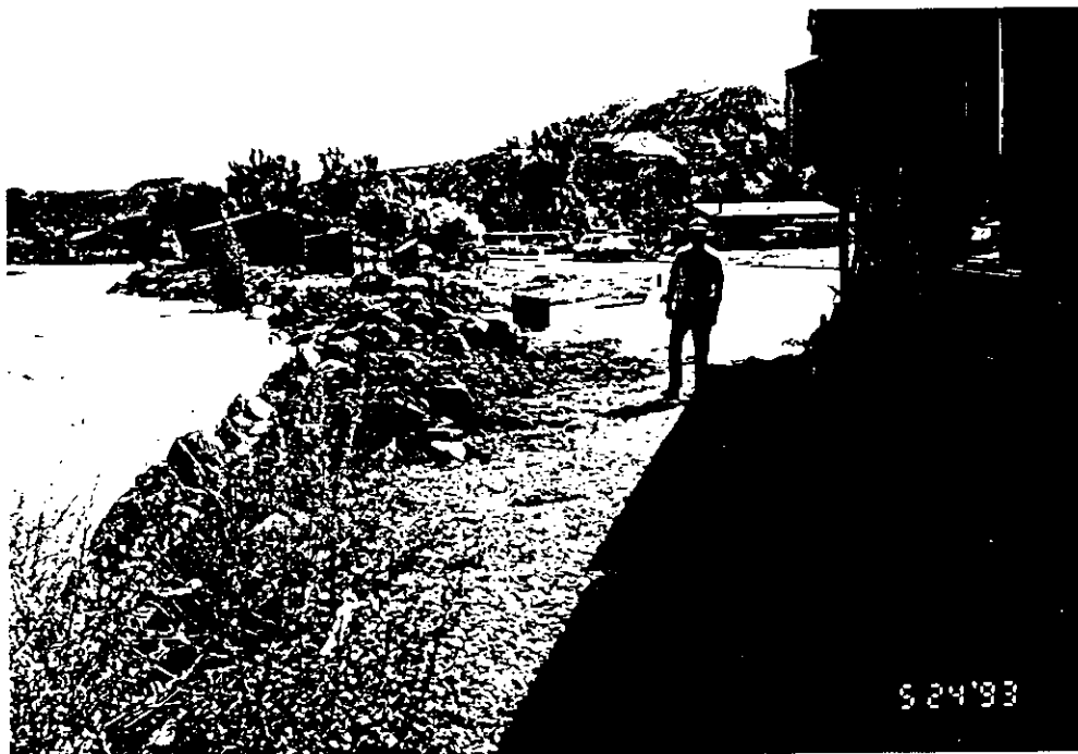
$5,000 Emergency Repair by Town of Paonia
