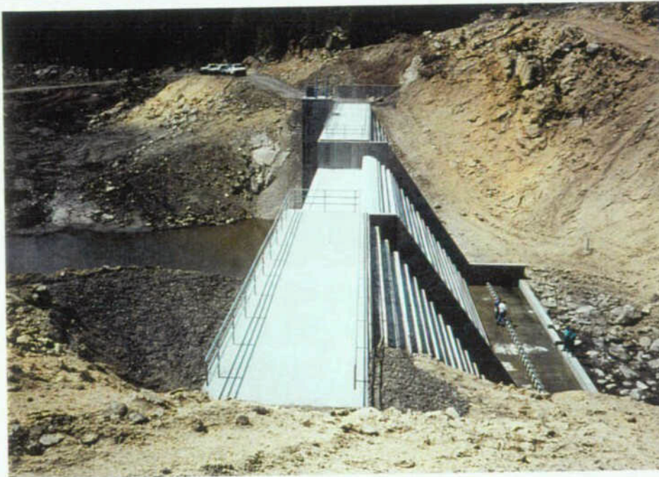
Looking North Along the Dam Axis Showing the Stairstep Spillway
