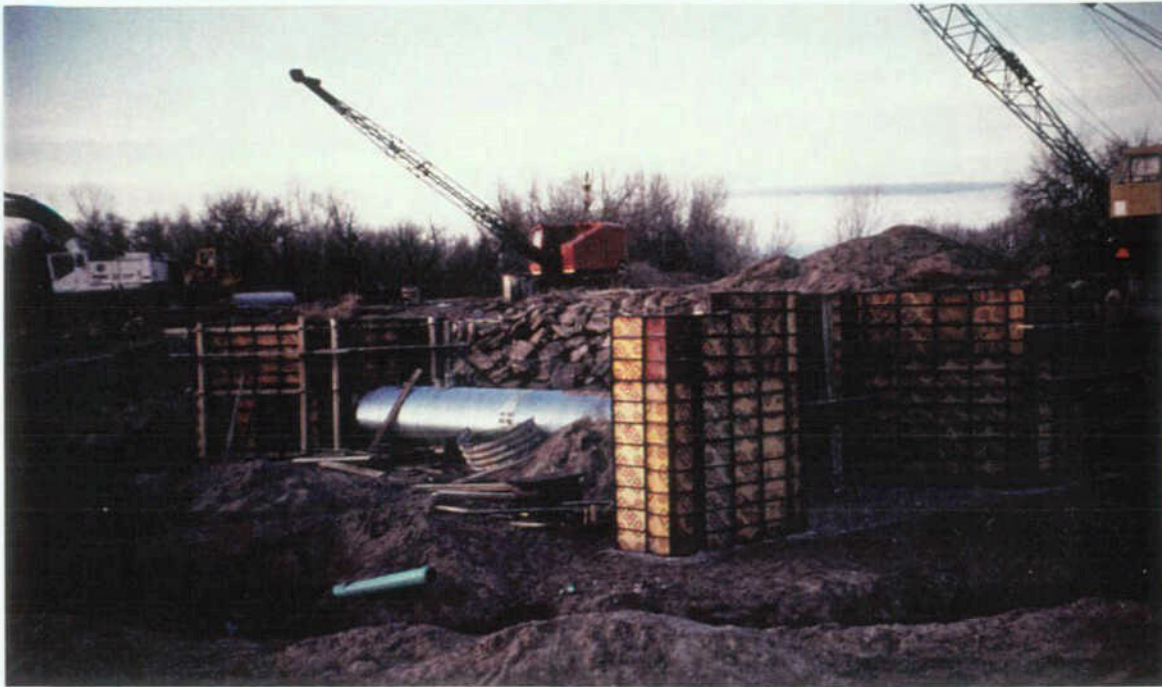
Headwall and Wingwall Forms Prior to Concrete Placement
