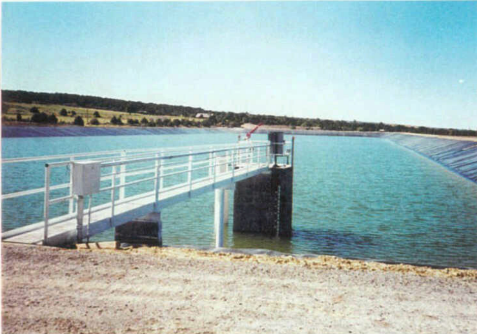
Looking West Past the Outlet Tower Bridge from the East Embankment
