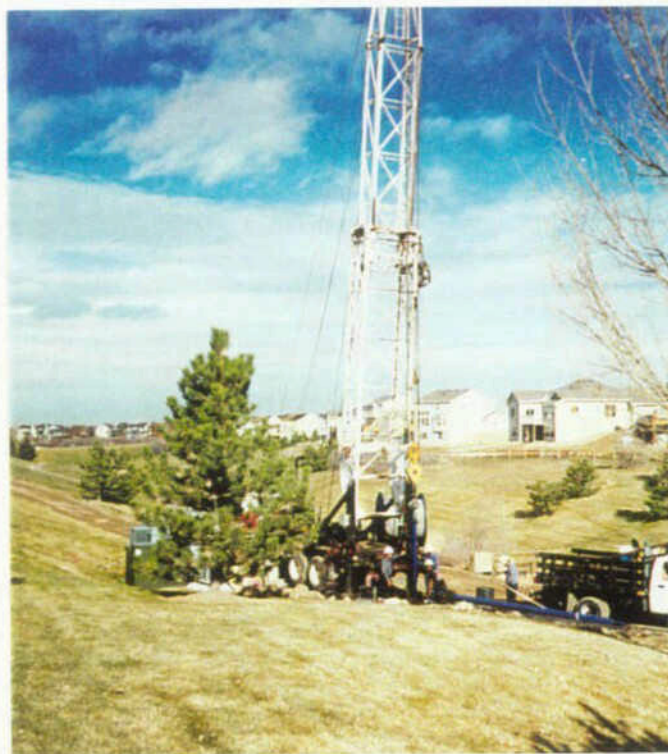
Brushing and Cleaning of Well A-2
