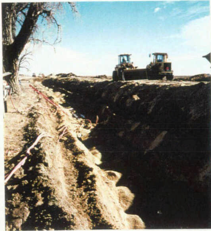
Excavated Pipeline Trench, Partially Backfilled
