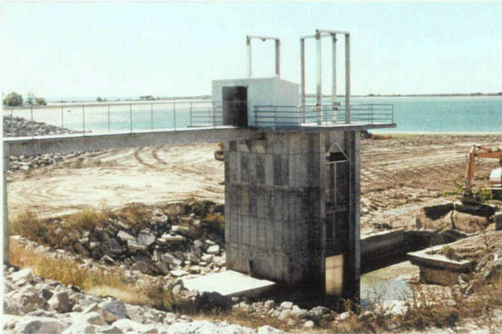
New Jumbo Reservoir Outlet Tower Looking West into the Reservoir
