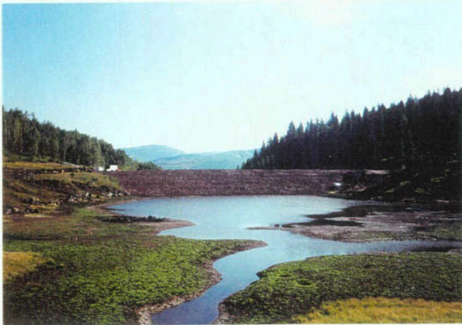
Looking North at the Upstream Face of Alsbury Dam from the Reservoir
