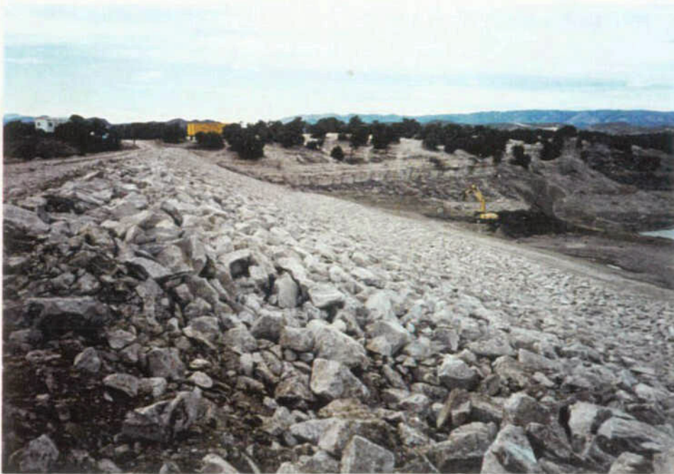
Stabilized Upstream Face of the Brush Hollow Reservoir Dam
