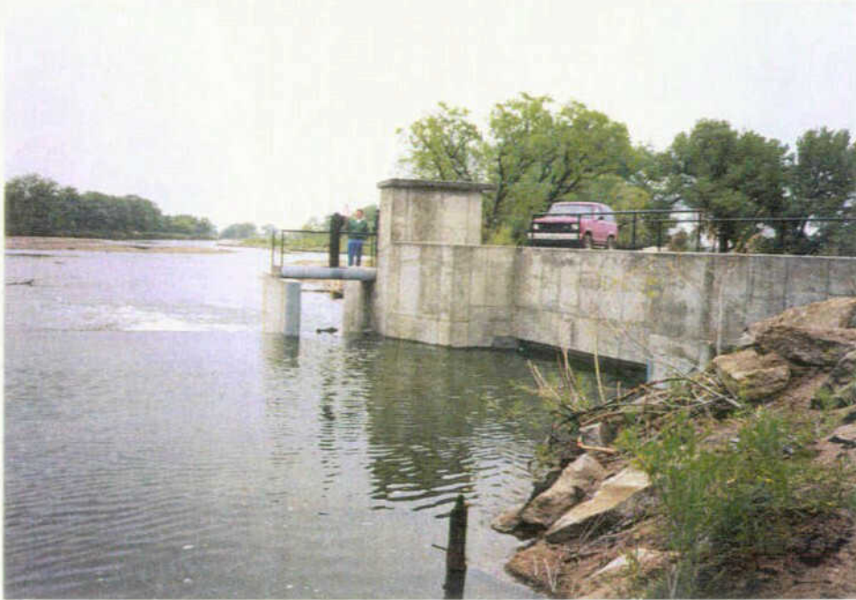
The Diversion Structure at the South Platte Ditch, Looking Downstream
