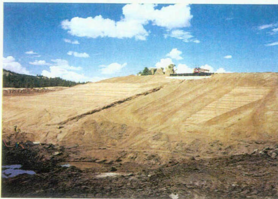
Upstream Face and Outlet Excavation of Worster Dam
