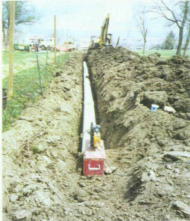
Trench Excavation and Pipeline Placement along the Rainbow Park Ditch
