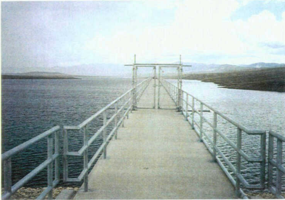
Looking West Into the Reservoir from the Dam's Outlet Tower Bridge
