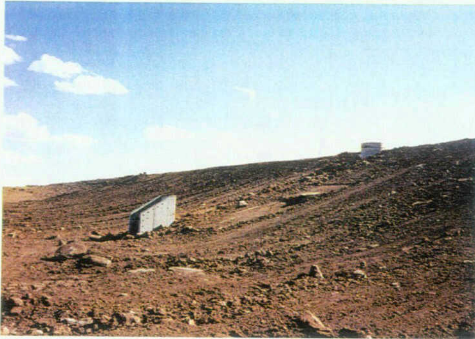
Rapid Creek Dam #2 Upstream Face and Outlet Intake
