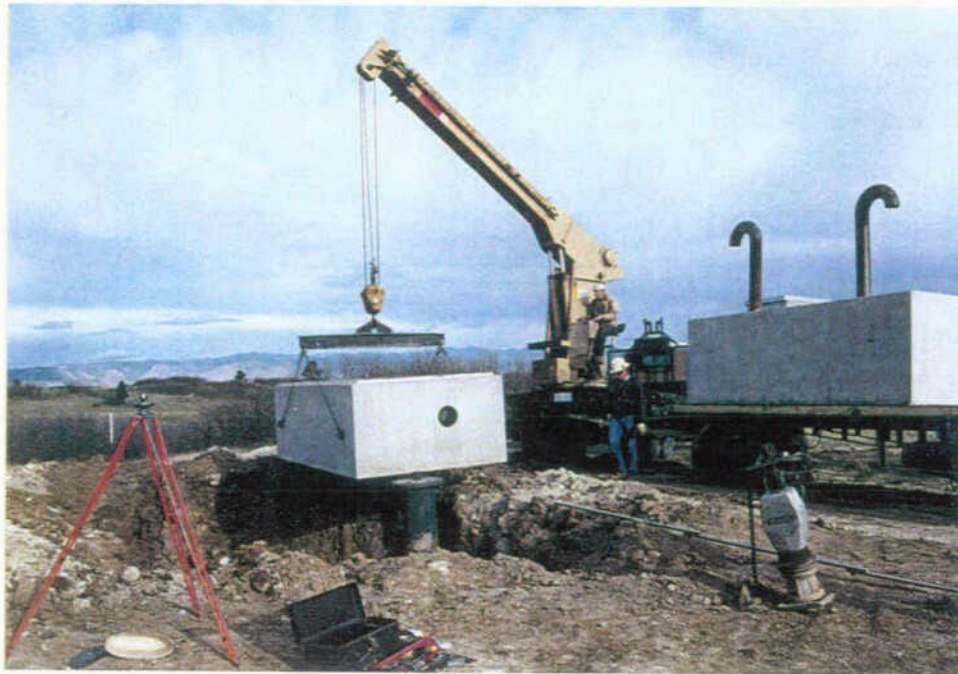
Placement of the Well Control Vault
