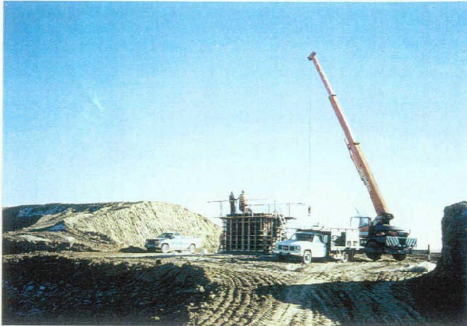
Re-construction of the North Poudre Reservoir #5 Outlet Tower
