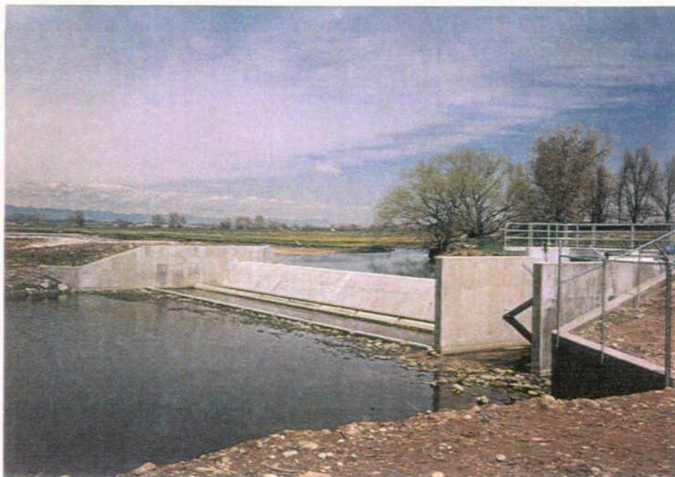
Downstream of the Diversion Structure Looking Upstream
