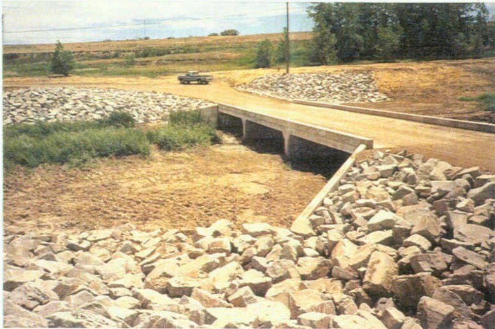
Cheeseman Street Low Water Crossing Looking From Top of Levee
