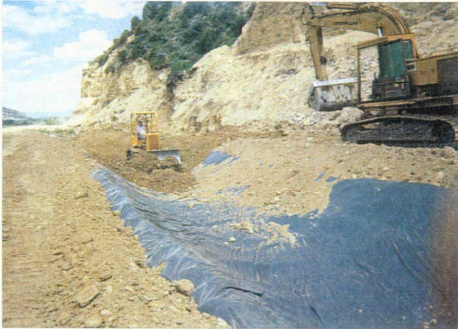
Placement and Backfill of the 30 mil Impermeable Geosynthetic Membrane Ditch Liner
