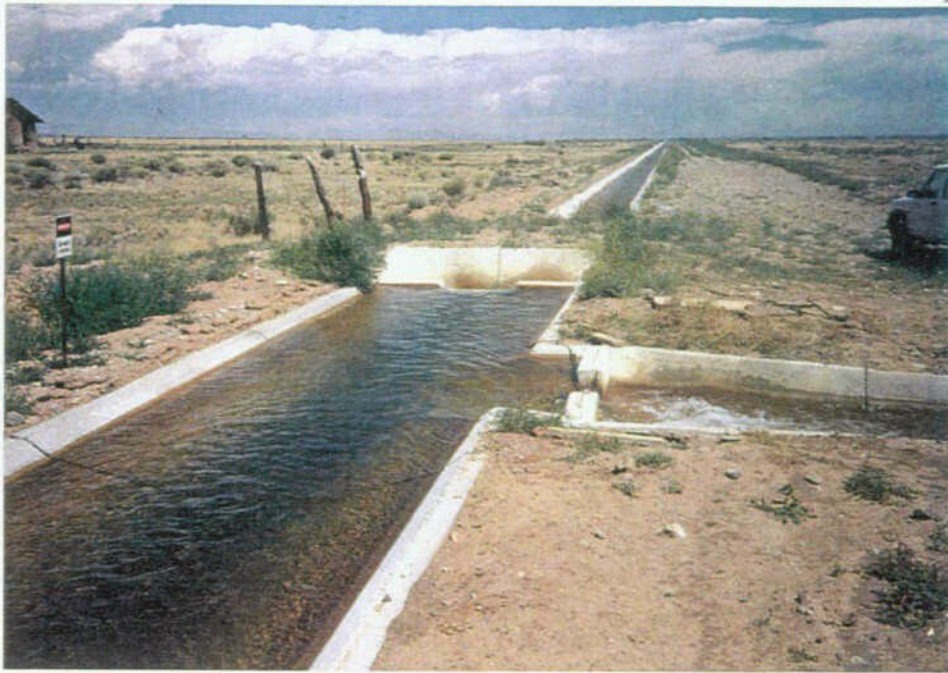
Alamosa Creek Canal Mainline looking North
