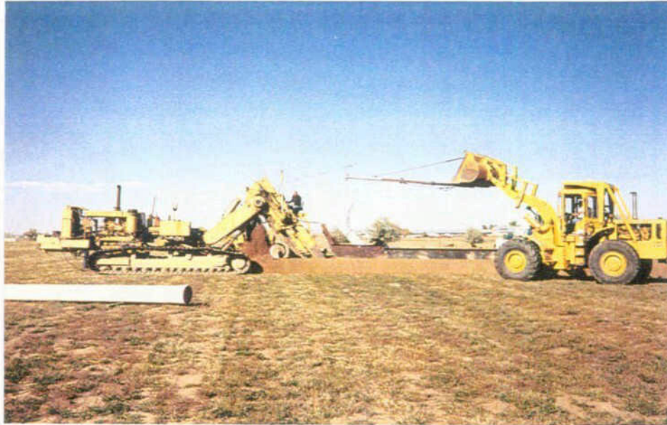
Placement of the 18 inch PVC Pipeline
