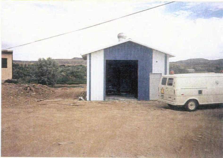
The Rangely Raw Water Intake Pump House looking north toward the White River
