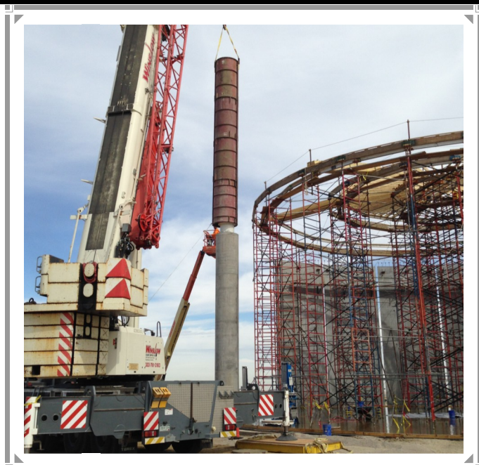
WISE project under construction—photo courtesy of SMWSA
