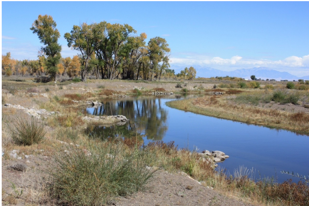
Rio Grande Riparian Stabilization Project — Phase 3
