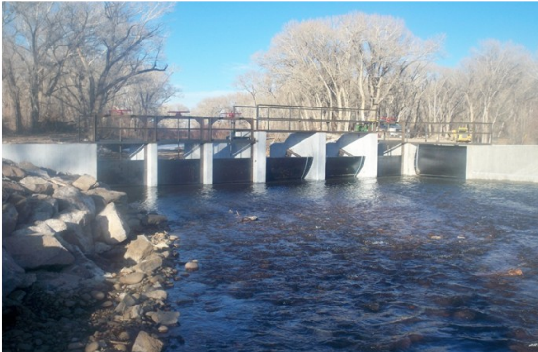
Manassa Land & Irrigation Company: Conejos River & North Branch Diversion & Stabilization Project
