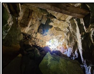
Unstable conditions inside the North tunnel.
