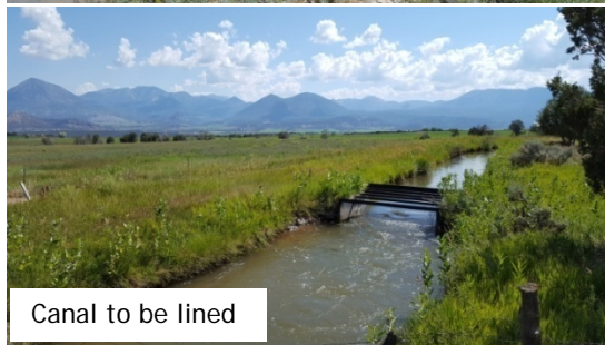
Canal to be piped
