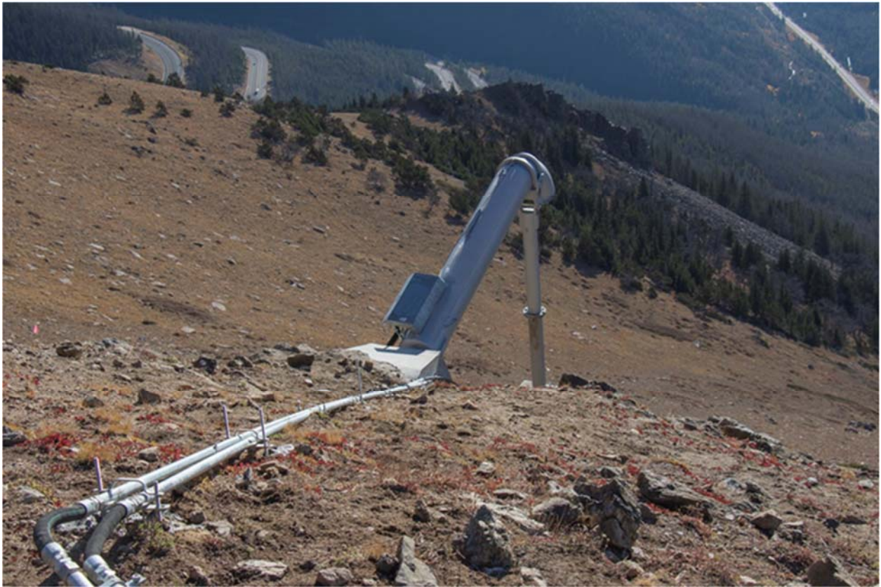
A Gazex exploder on Berthoud Pass above US40. Gas flows from a storage shelter through the pipes in the foreground and into the large gray pipe, or exploder. There it ignites, creating a blast that releases an avalanche on the open slope.
