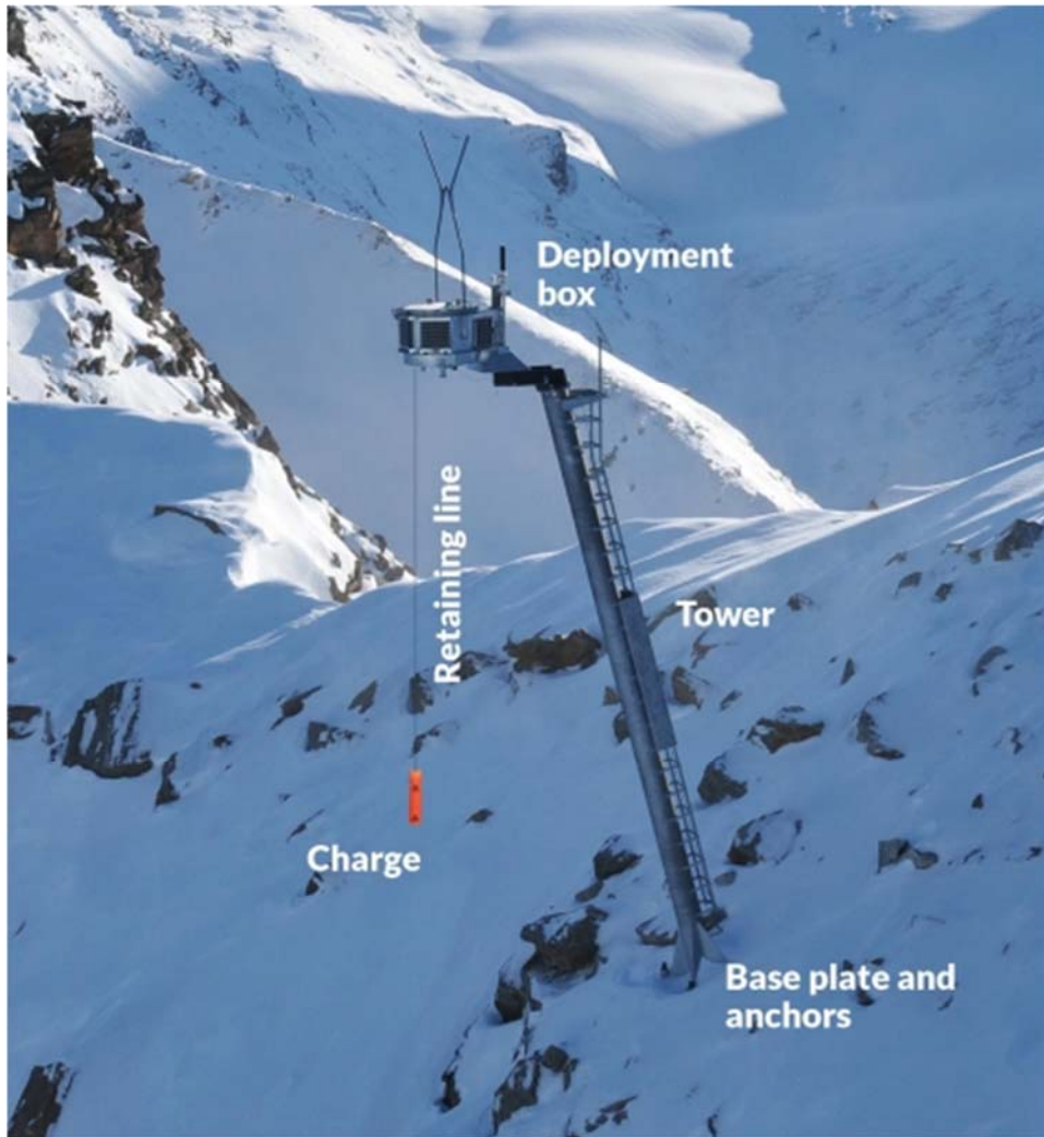
A Wyssen Avalanche Tower LS12-5 remote avalanche control system (RACS). The deployment box containing a set of explosive charges is delivered to the tower by helicopter. Avalanche crews release each charge during periods of high avalanche hazard. The box is retrieved and reloaded each fall. (Image courtesy of Wyssen Avalanche Control)
