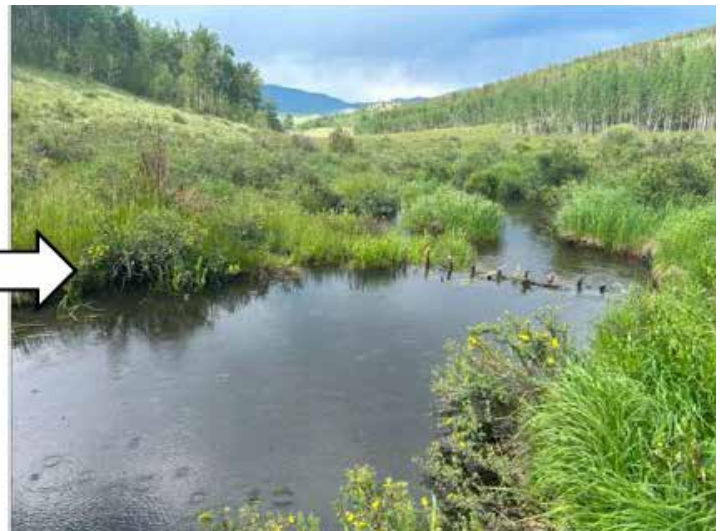
Pre- and post-restoration images of the Kenosha Creek Restoration project. This project used low-tech, process-based restoration techniques (including beaver dam analogs) to reconnect an incised stream to its floodplain. ©Colorado Open Lands/EcoMetrics
