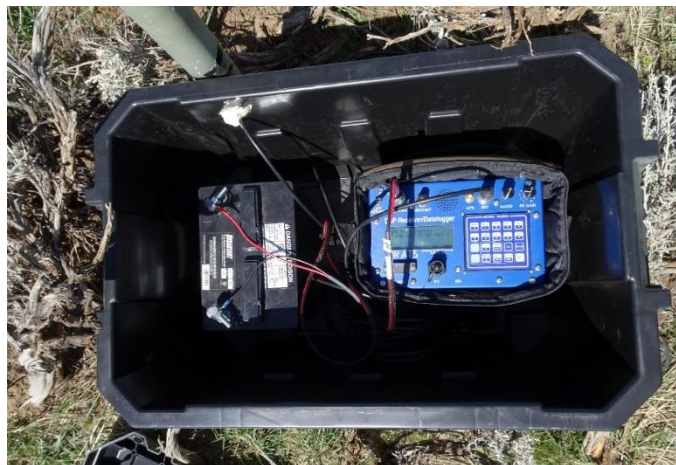
Figure 8. An Advanced Telemetry Systems datalogger connected to the 12-volt battery inside the waterproof box in the Axil Basin area of Moffat County, Colorado, 2018.
