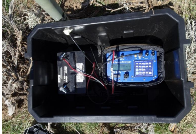
Figure 3. The ATS datalogger connected to the 12-volt battery inside the waterproof box on the SG4/Collom 2 lek in northwestern, Colorado.
