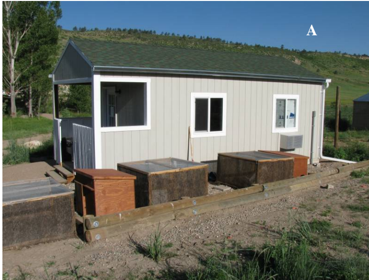
Figure 3. CPW Foothills Wildlife Research Facility incubation building. In February, 2010, we built a facility (A) to house all of the egg incubation and hatching operations. The building allowed us to better control temperature and humidity as well as have a clean work space to help prevent bacteria growth. The building is 3.7-m x 6.1-m x 2.4-m (W x L x H). The building electricity was wired to have separate breakers for each of the incubators and hatchers (B). The building also had a heating and air conditioning unit as well as a sink and water heater. Brooder pens and coops (A) were also provided at the facility.
