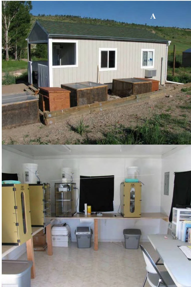
Figure 6. CDOW Foothills Wildlife Research Facility incubation building. In February, 2010, we built a facility (A) to house all of the egg incubation and hatching operations. The building allowed us to better control temperature and humidity as well as have a clean work space to help prevent bacteria growth. The building is 3.7-m x 6.1-m x 2.4-m (W x L x H). The building electricity was wired to have separate breakers for each of the incubators and hatchers (B). The building also had a heating and air conditioning unit as well as a sink and water heater. Brooder pens and coops (A) were also provided at the facility.
