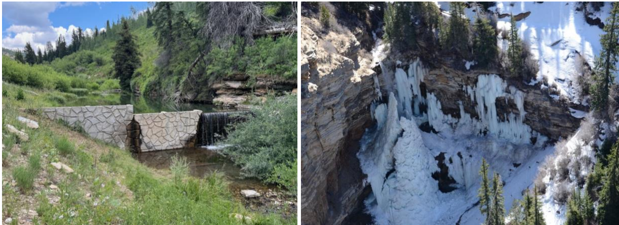
Figure 1. The temporary concrete barrier that bisects the headwaters of E Fk Parachute Creek is shown on the left, while the stream drops over the East Fork Falls from the top left of the right photograph.
