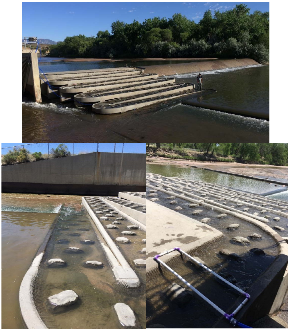
Figure 11. Fish passage structure on the Owens-Hall Diversion, Fountain Creek, Colorado.
