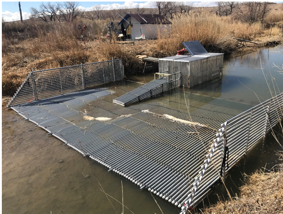
Figure 3. The fully assembled resistance board weir (RBW) in Roubideau Creek. The photo faces upstream. The PVC pickets in foreground are anchored on the upstream end to a substrate rail, but can pivot freely with water level. The only passage through which fish can pass is the PVC chute leading into the aluminum cage. The wall-tent in the back ground houses the fish-working station.
