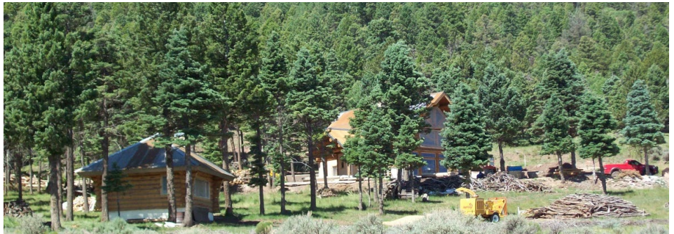
Landowners can reduce their risk of wildfire by removing flammable materials, such as dead and dying trees or dense woody material, near their homes and other structures. Photo: CSFS
