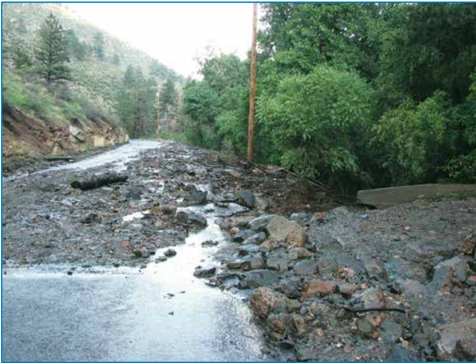
▲ Due to the loss of vegetation after the High Park Fire in Larimer County, heavy rains caused extensive sediment and debris flow into streams and rivers in the burn area. Photo: Tony Simons, Larimer County Emergency Services
