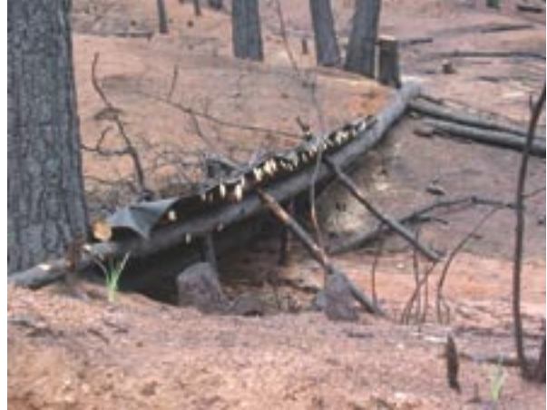
13. Silt fence on Hayman Fire site.
