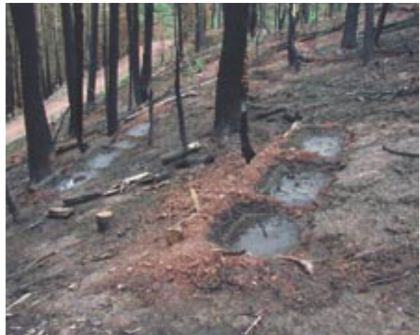
12. Erosion barrier created from a burned log.
