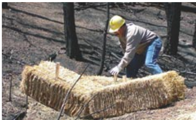
15. A rehabilitation worker puts straw bales in place to slow post-fire erosion.
