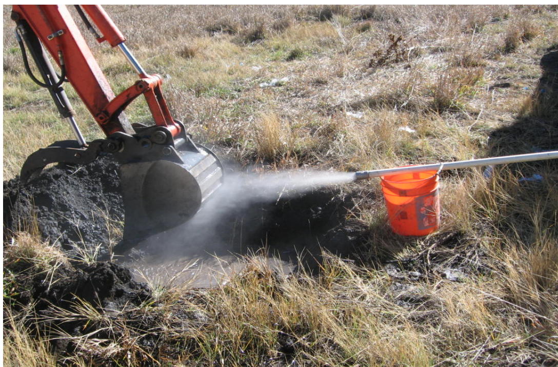
Figure 7. Air-lift discharge from MW 35-7-8-2 diverted into containment pit.
