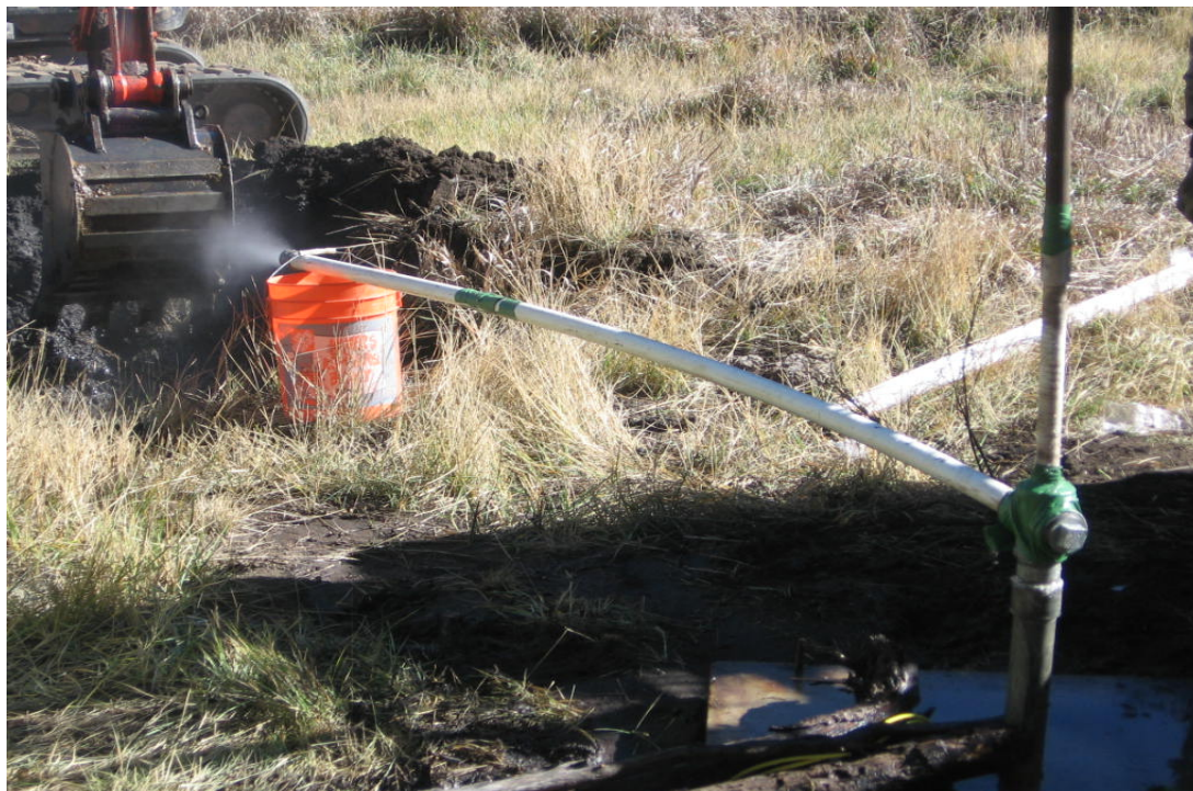
Figure 6. Air-lift apparatus used to development of MW 35-7-8-2.
