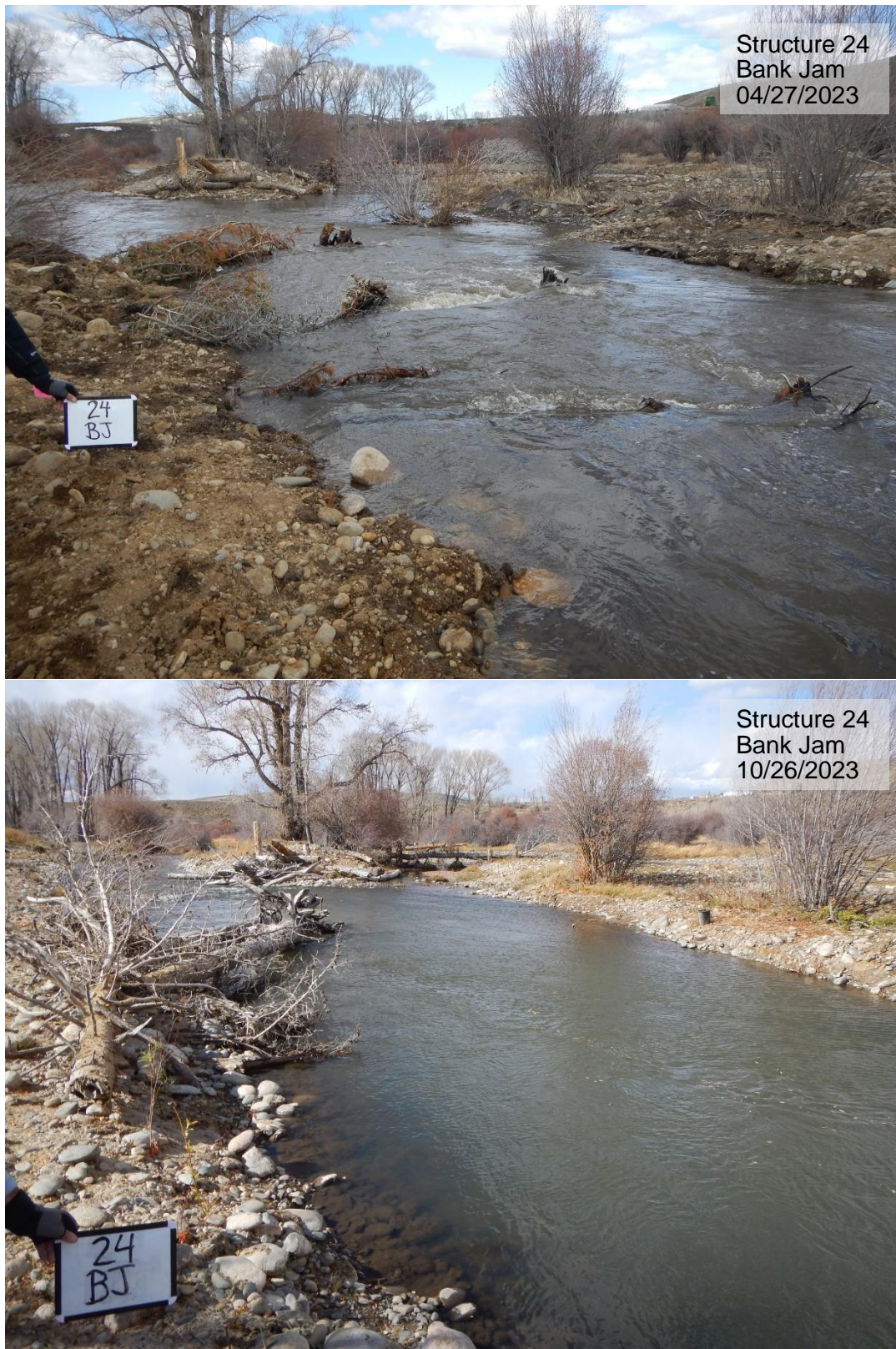
Figure 12. Example of failed bank-jam structure from log-jam assessments at the Kemp-Breeze SWA Habitat Project on the Colorado River.
