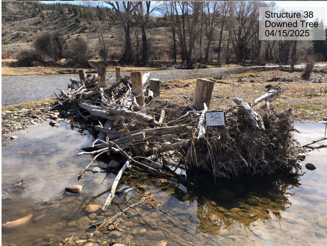
Figure 13. Example of wood racking on a downed cottonwood tree from log-jam assessments at the Kemp-Breeze SWA Habitat Project on the Colorado River.
