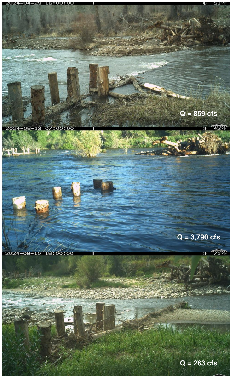
Figure 11. Select photos showing flows (Q) in the Phase 2 project reach of the Kemp-Breeze SWA Habitat project during 2024, including a downed cottonwood tree in the foreground, as well as a gravel augmentation pile, constructed island, and bar-apex jam in the background.
