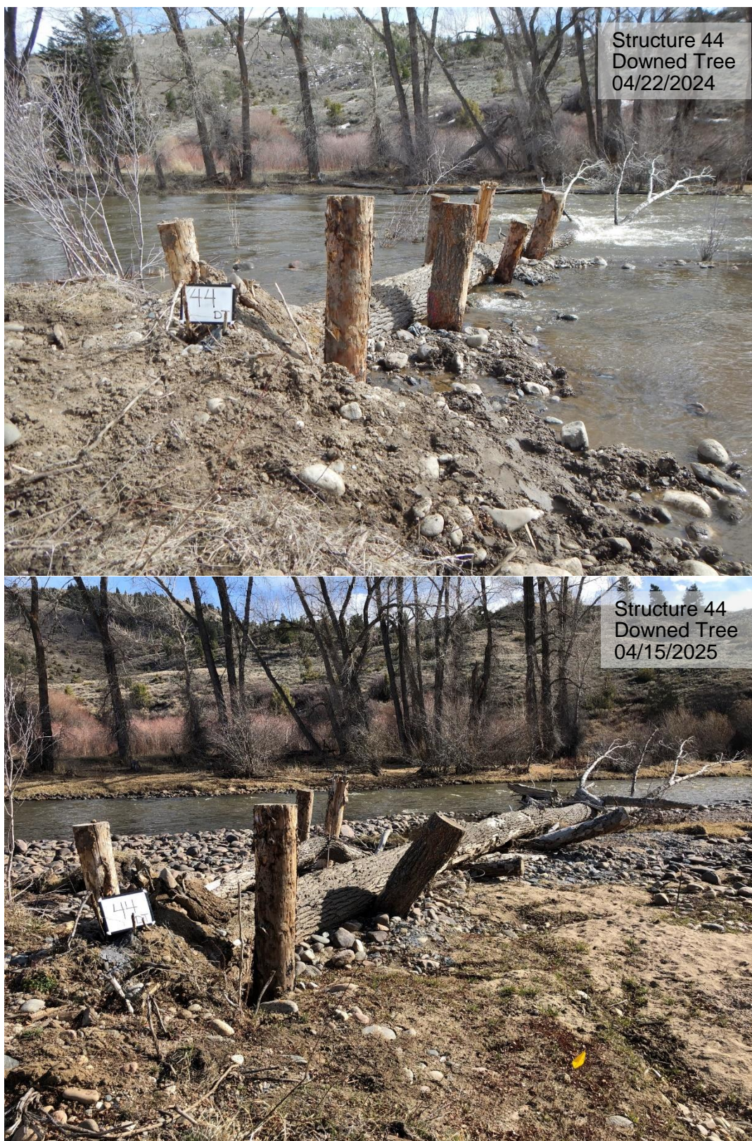
Figure 14. Example of failed piles at a downed cottonwood tree observed during log-jam assessments at the Kemp-Breeze SWA Habitat Project on the Colorado River.
