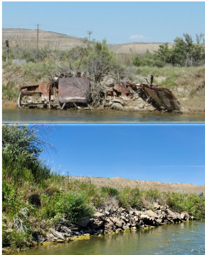
Figure 19. Bank stabilizing techniques typical of the White River downstream of Meeker, Colorado, including use of car bodies and concrete rubble.
