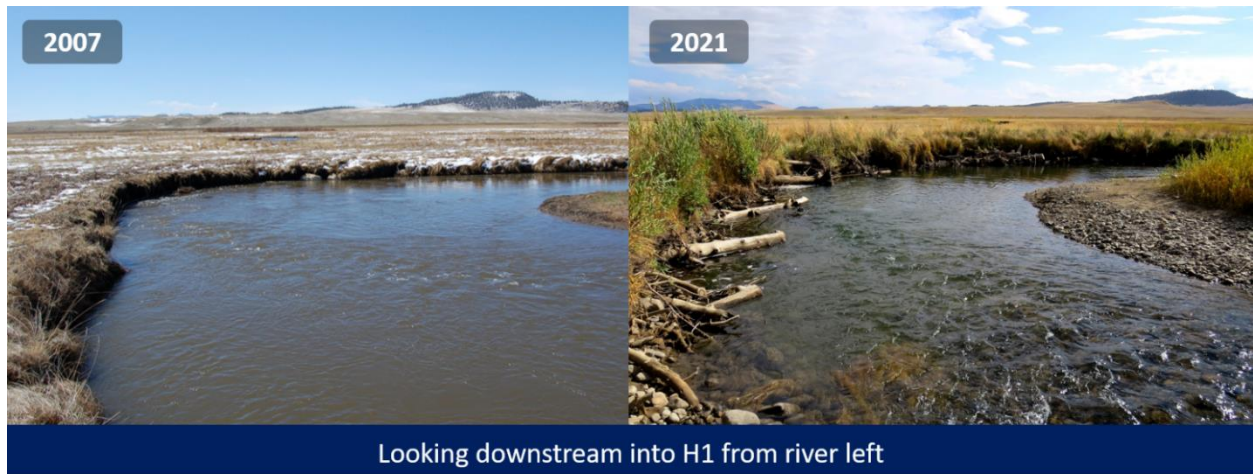
Figure 15. Photos showing riparian vegetation and bank conditions before (2007) and after (2021) construction at a haphazard toe wood-treated pool site. Note differences in deep-rooted willow abundance, large wood presence, and coarseness of sediments composing the streambed and point bar in before versus after photos.
