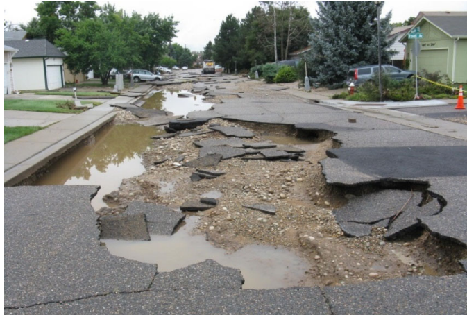
Figure 7: Damage to Hayden Court, Longmont (Source: Survey)
