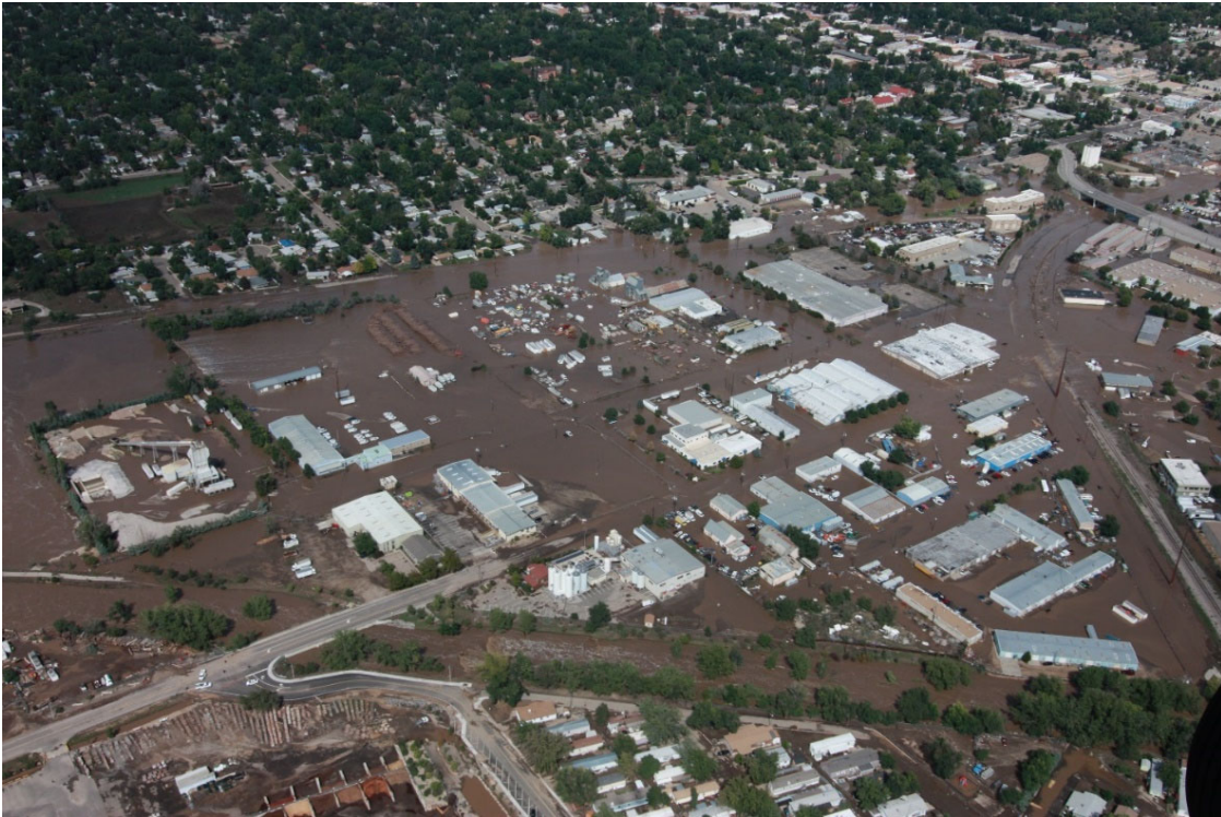
Longmont St. Vrain Creek Flooding, September 2013
