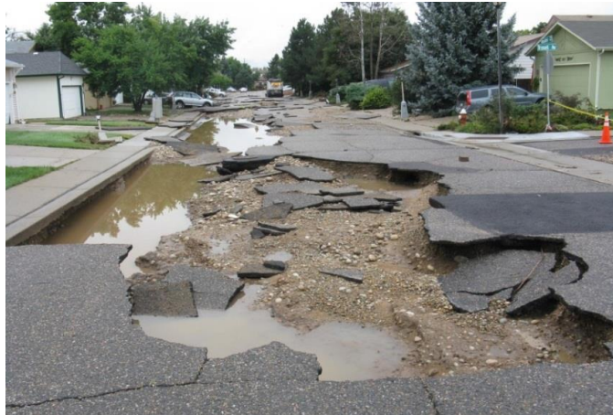
Figure 7: Damage to Hayden Court, Longmont (Source: Survey)
