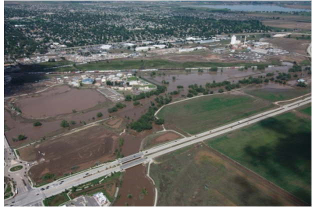
Figure 4: Longmont Wastewater Plant (Source: Survey)
