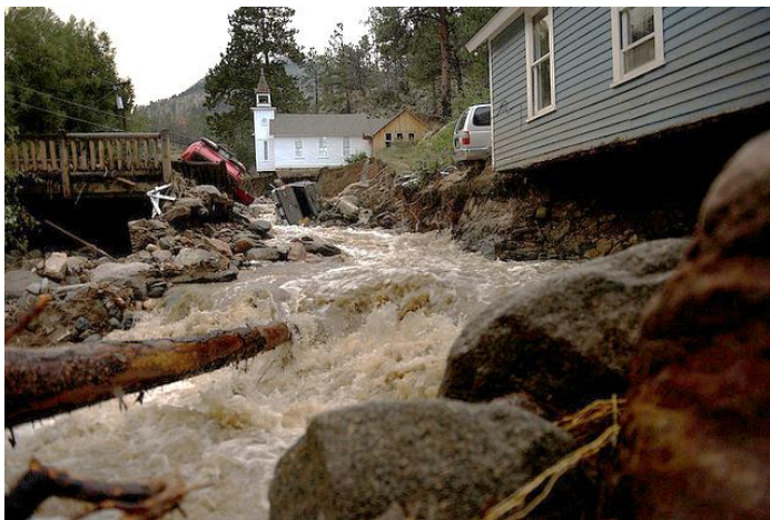
Figure 1: Damage in Salina (Source: Boulder Co.)
