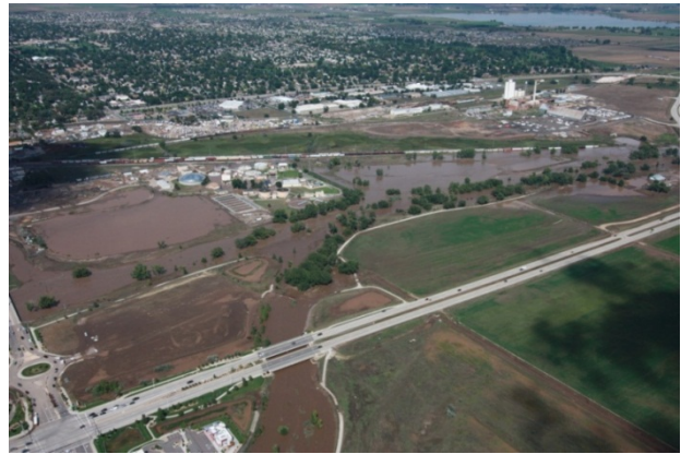
Figure 4: Longmont Wastewater Plant (Source: Survey)
