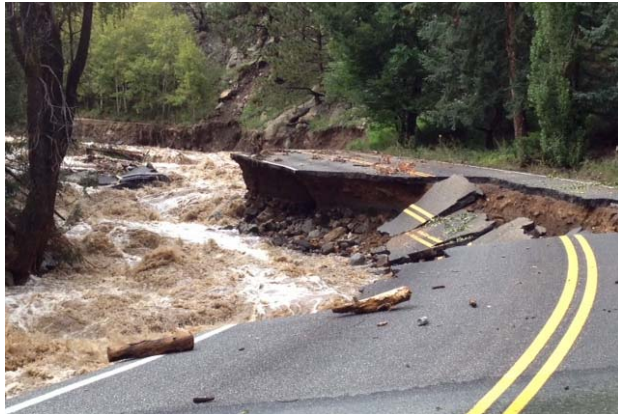
Figure 3: Fourmile Canyon (Source: Boulder Co.)
