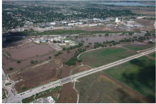
Figure 4: Longmont Wastewater Plant (Source: Survey)
