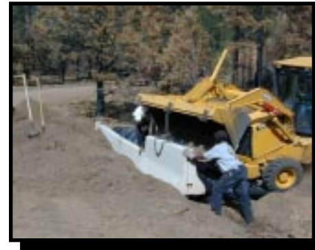
Culvert barrier being installed in the Hayman Burn Area.
